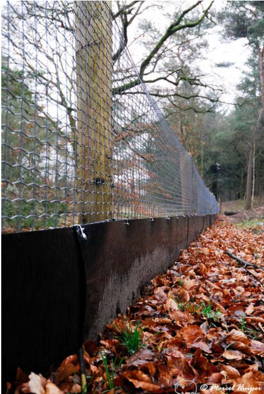
Figure 23: Wildlife fences including smooth plastic amphibian screen, N302, Leuvenumseweg, Sonnevank, east of Harderwijk, The Netherlands.
