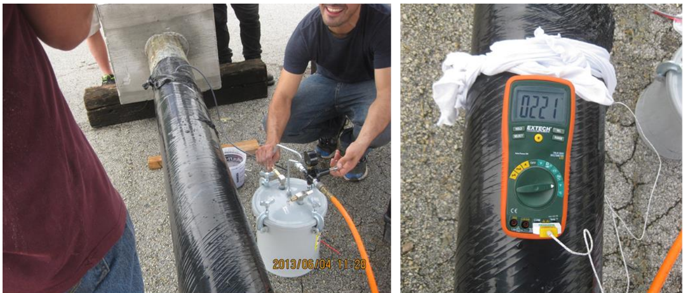
Figure 4.7: Injection of pre-mixed resin using a pressure pot
