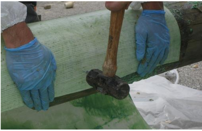
Figure 4.4: Wrapping GFRP sheet around the pile
