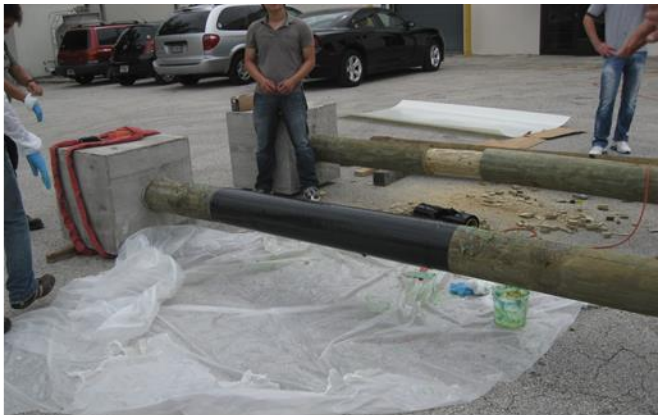
Figure 4.5: Holding GFRP sheet around the pile by Saran™ plastic wrap
