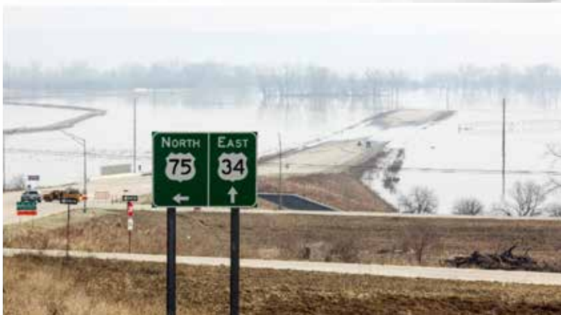
Flood damage near the Hwy 34/75 intersection at La Platte.
