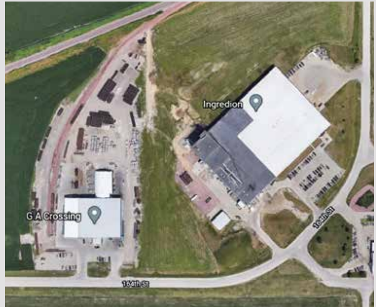
South Sioux City and Ingreion Company's completed rail spur.
