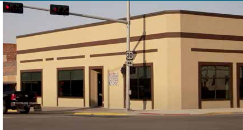
The newly renovated building is no longer a blight on downtown Kimball. Photo Credit: Olsson Associates
