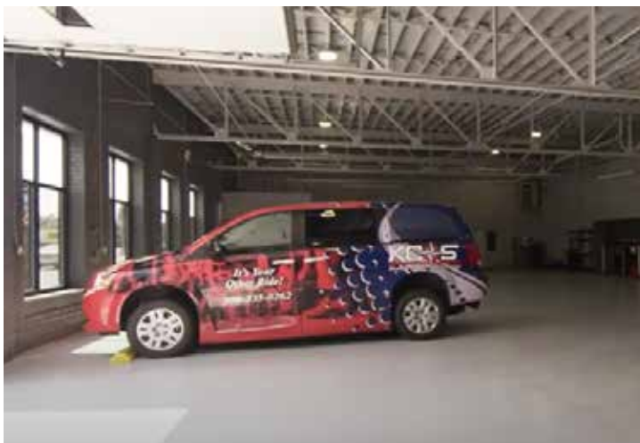
The facility includes a garage to house 12 federally funded transit vehicles and a wash bay. Photo Credit: Olsson Associates
