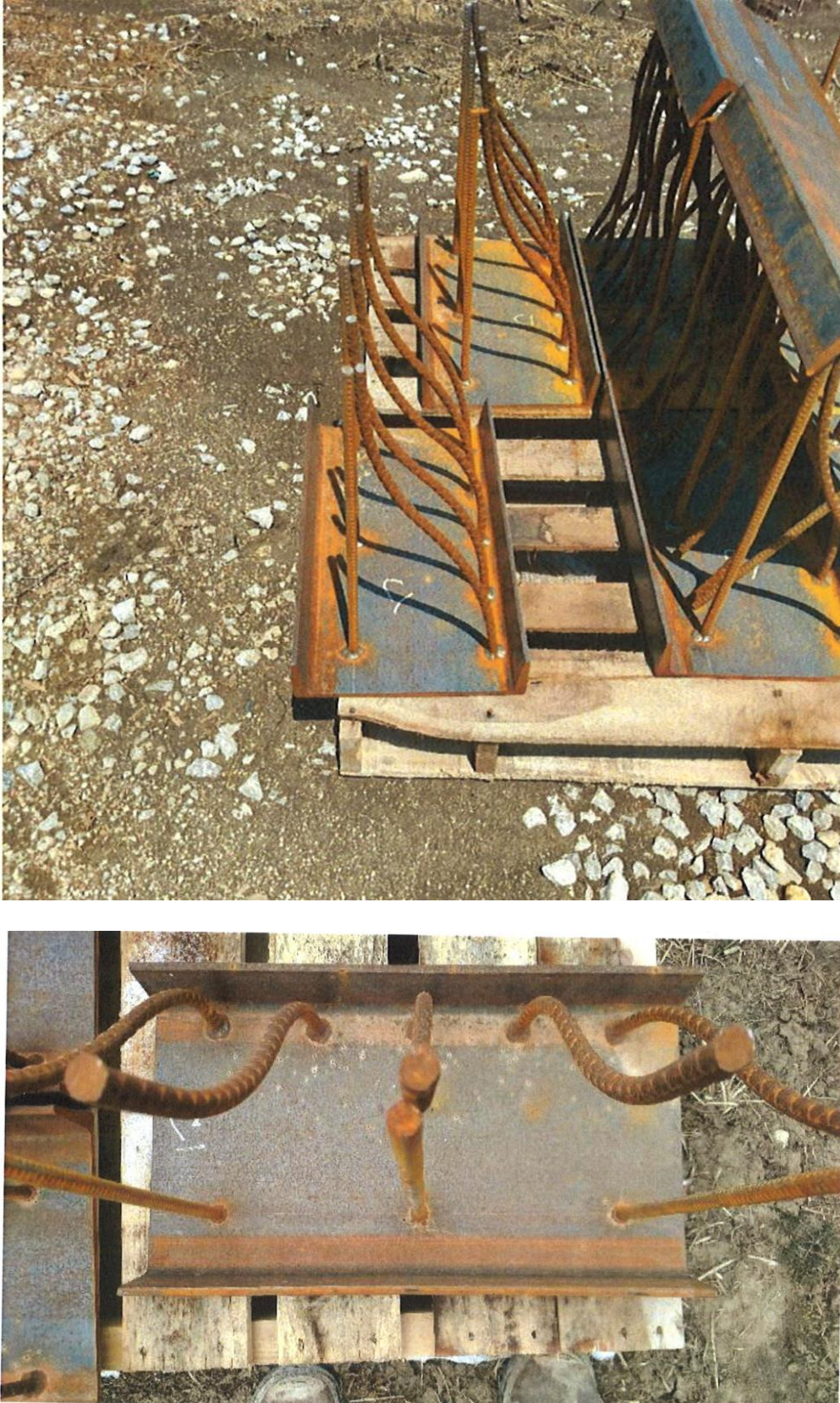
Figure 5. Short Channel Segments Used Within a 12-in. Thick Beam-Slab Deck
