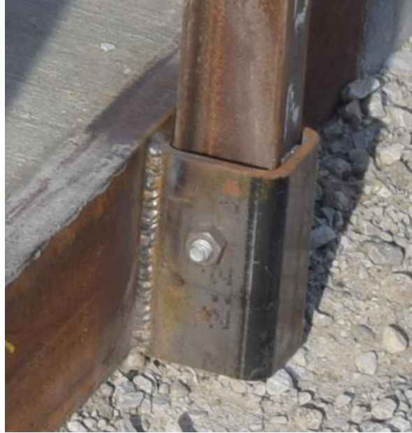
Figure 8. Socket Welded Directly to a 7-in. CIP Deck
