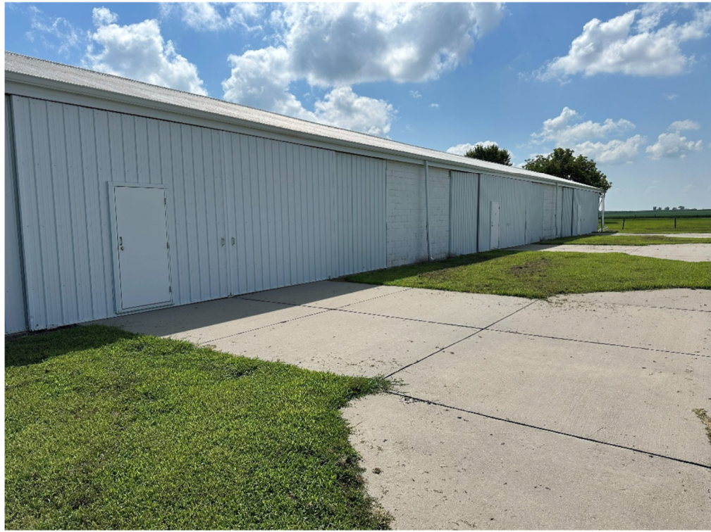
Figure 3 – Second T-Hangar constructed at Brenner Field
