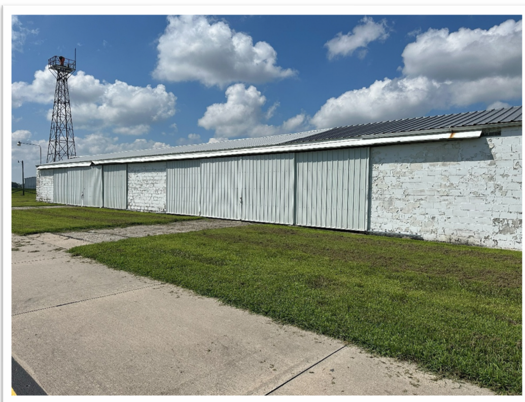
Figure 2 – The original T-Hangar building at Brenner Field.
