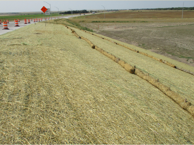
Pictured: Good Erosion Control Blanket installation.
