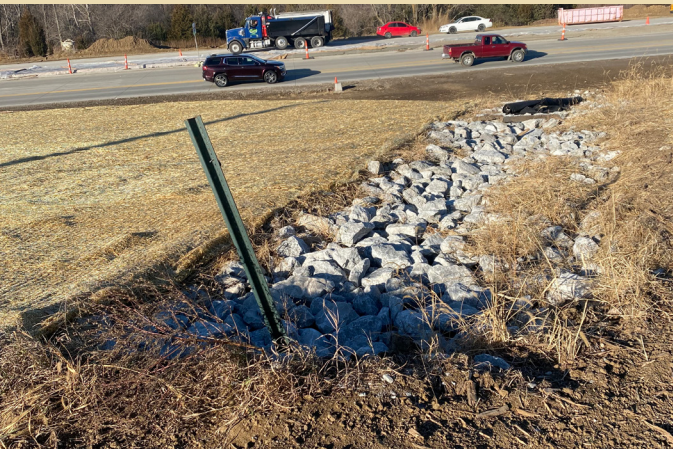
Pictured: Outlet is protected with riprap and adjacent areas are mulched and seeded to prevent erosion. Additional barriers around outlet could prevent sediment from getting into the channel until final stabilization is established.
