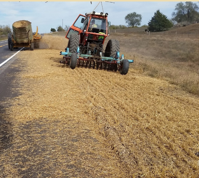
Pictured: Good installation of mulch
