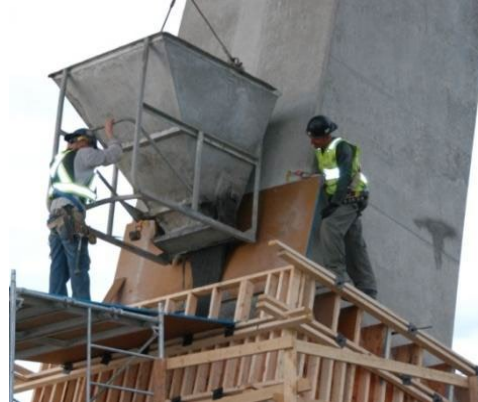
Figure 2.4 Casting UHPC jacket around bridge pier using hopper (Doiron, 2017)
