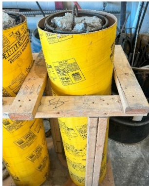
Figure 4.19 Supportive skeleton for the form work
