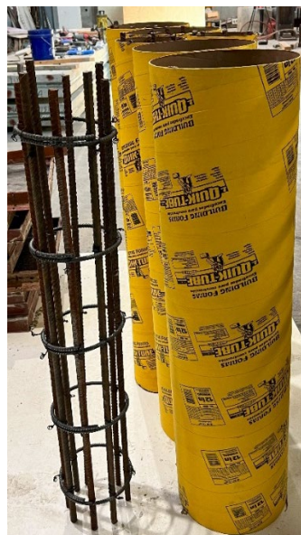
Figure 4.13 Steel cage of column and the concrete tube form
