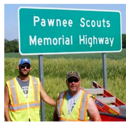
NDOT District 4 Highway Maintenance Workers Adam Bialas and Paul Glup install the Pawnee Scout Memorial Highway signs, along Hwy. 22, one near Genoa and the other near Fullerton.
