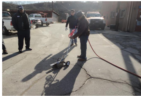
(c) Testing by GDOT crew
