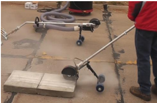
Figure 3.3 Creating saw joints on concrete
