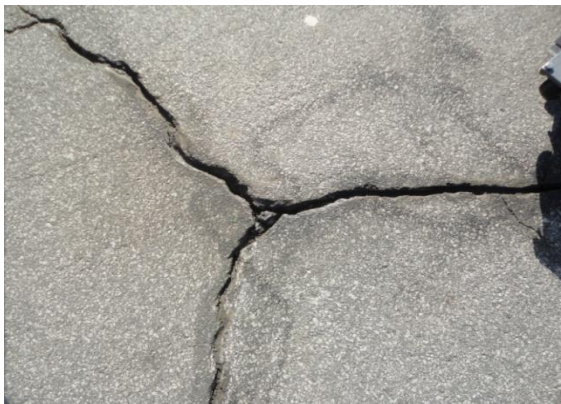
(b) Routed cracks
