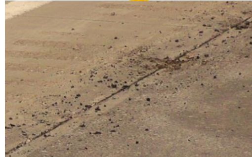
(b) Router : Cleaned crack, requiring a separate application for air blowing
