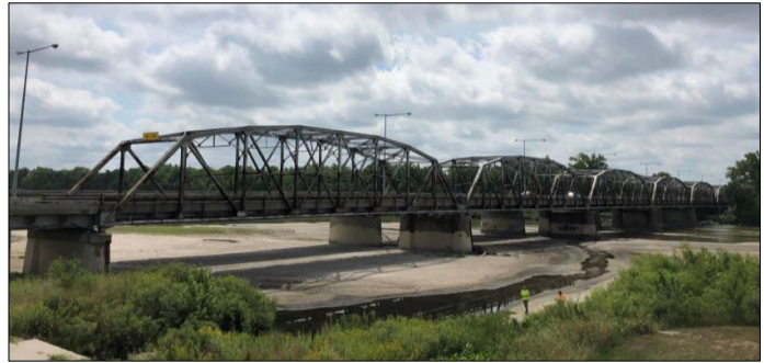
Figure 3. The historic Columbus Loup River Bridge, now no longer extant.
