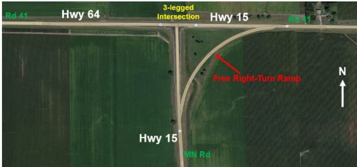
Figure 7.1 Three-Legged One-way Stop-Controlled Intersection with FRT Ramp at Bone Creek, Nebraska (Location coordinates: 41.333405, -97.129290)
