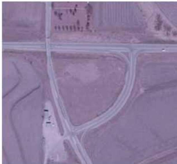
Example of One-Quadrant Interchange (Intersection of US 59 and US 34 in Mills County, Iowa)
