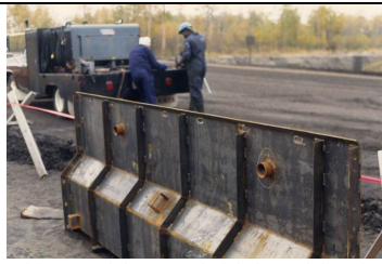
Figure 17: Patching steel formwork fabricated for girder restoration, AIT, 2005
