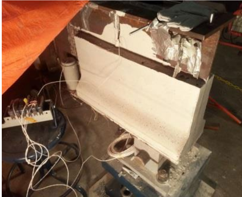
Figure 57: UHPC encasement at the repaired girder end zone, courtesy of Zmetra, 2015
