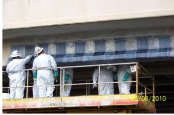
Figure 22: FRP wrapping, CFRP confinement of patch, Harries et al., 2012
