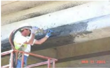
Figure 19: Shotcrete patch, Harries et al., 2012
