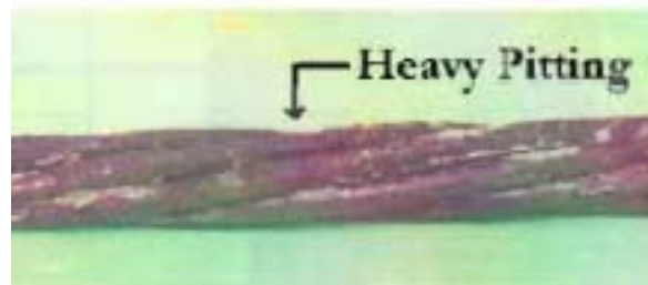
Figure 8: Severe damage, exposed strands having corrosion with heavy pitting, Naito et al., 2006
