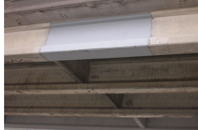
Figure 23: FRP Wrapped Repair, Iowa Dot, 2014
