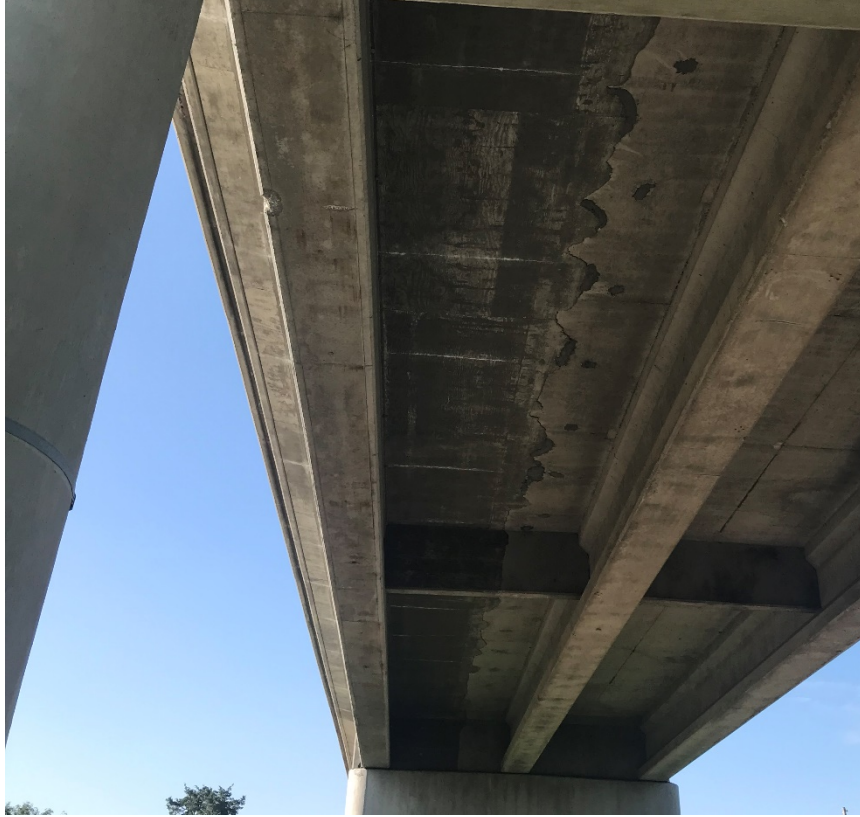
Figure 96: Replaced girder, York East Bridge, courtesy of NDOT
