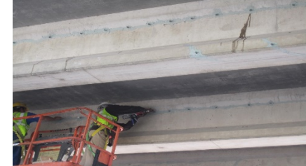
Figure 21: Epoxy injection process done in I-680 over US-75 Bridge
