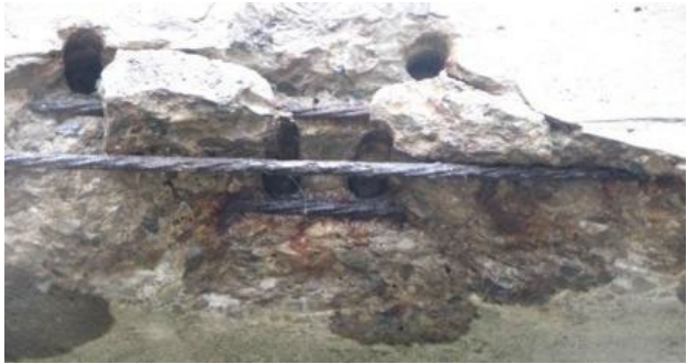
B: Exposed strands without corrosion
