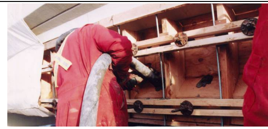
Figure 18: Pumping concrete into plywood formed section, AIT, 2005
