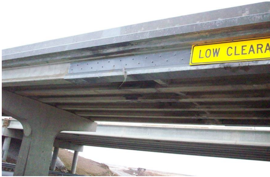
Figure 35: Grouted steel sleeve repair, courtesy of Iowa Dot, 2014
