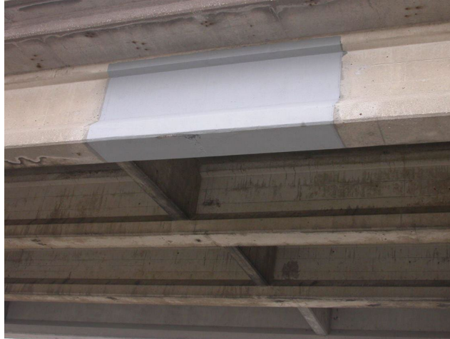
Figure 34: FRP Wrapped Repair, courtesy of Iowa Dot, 2014
