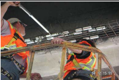
Figure 28: Strand splicing with a torque wrench, Enchayan, 2010
