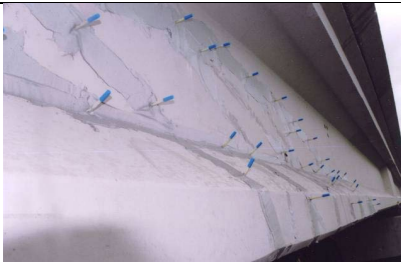
Figure 16: Epoxy injection ports, AIT, 2005
