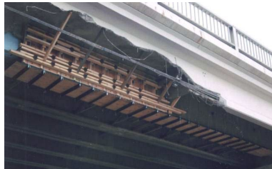
Figure 20: Patching plywood form to restore cross-section, AIT, 2005
