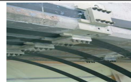
Figure 30: Sika carbon stress system external CFRP post-tensioning, Kasan, 2009
