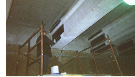
Figure 24: CFRP fabrics installation, Choo et al., 2013
