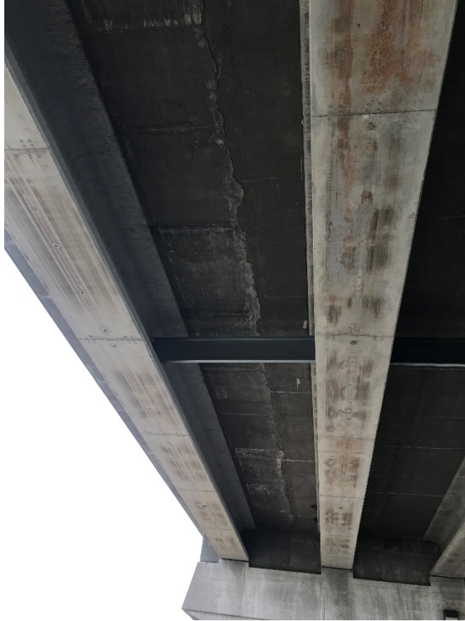
Figure 73: Replaced girder with no notable deficiencies, Schuyler Bridge, courtesy of NDOT
