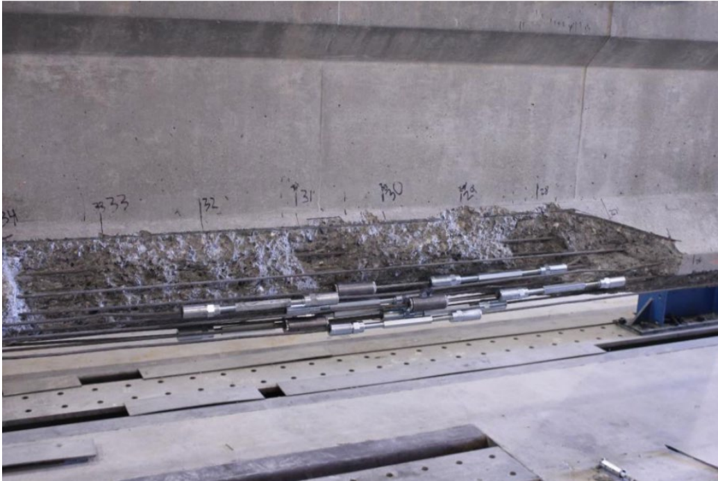
Figure 29: Strand splicing, courtesy of Jones, 2017
