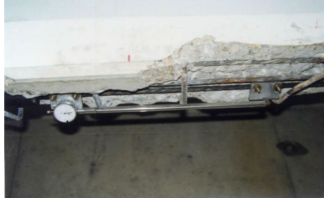
Figure 26: Strand splicing, dial gauges and devices to monitor elongations and strand force, AIT, 2005
