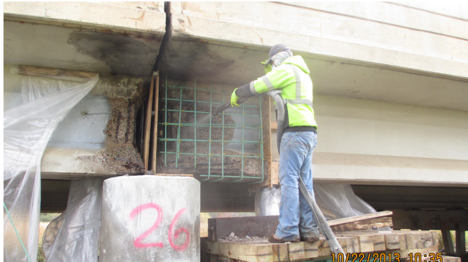
Figure 51: Shotcreting repair at girder end, MN/RC 2018-07 Report
