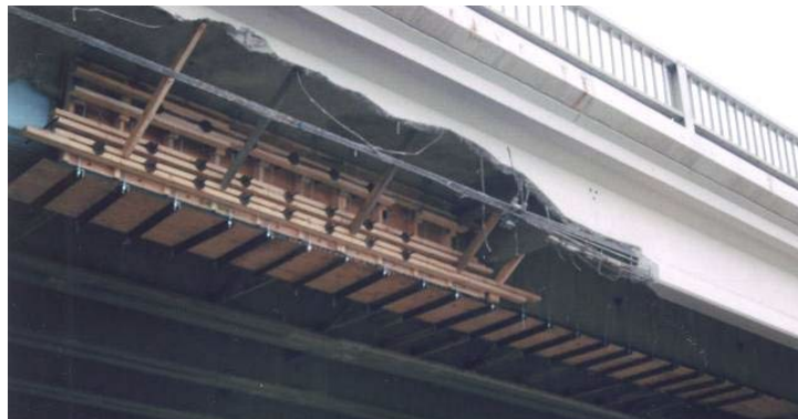
Figure 27: Patching formwork around girders, courtesy of Alberta Infrastructure and Transportation, 2005
