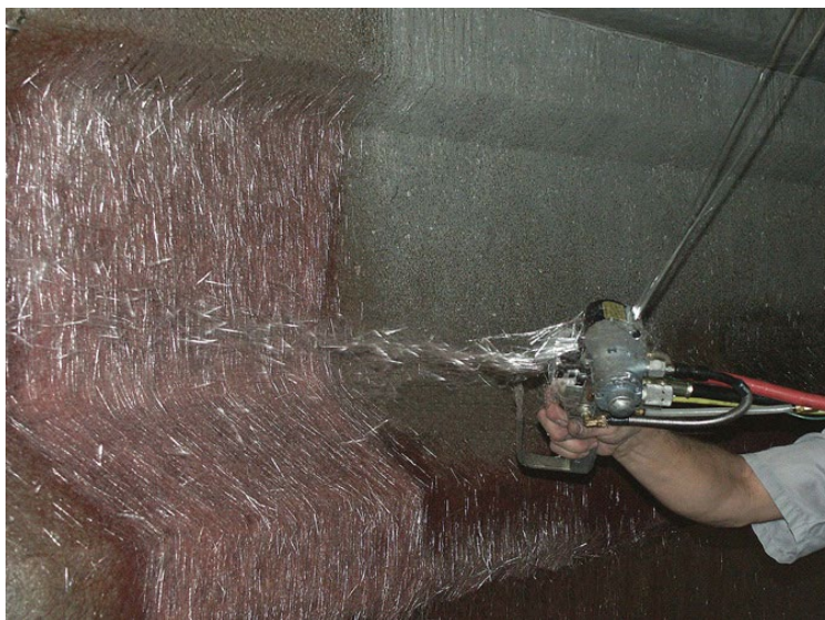
Figure 36: Sprayed GFRP technique, courtesy of Boyd et al, 2006
