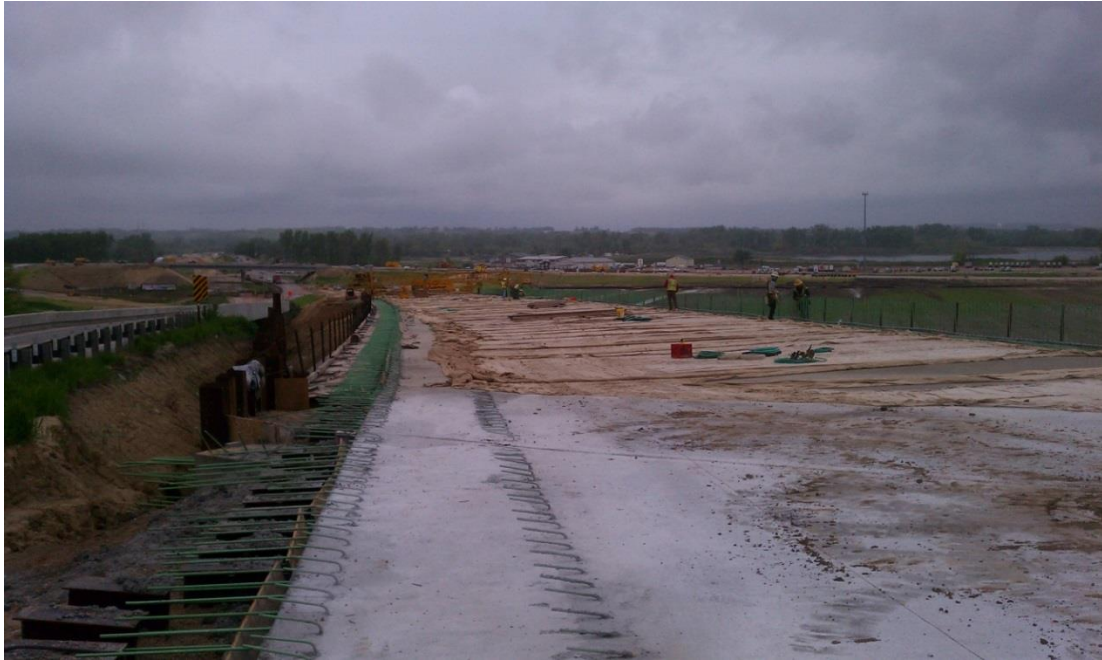
Figure 5.2 Phase 1 – Concrete Cure Process (May 22, 2013)
