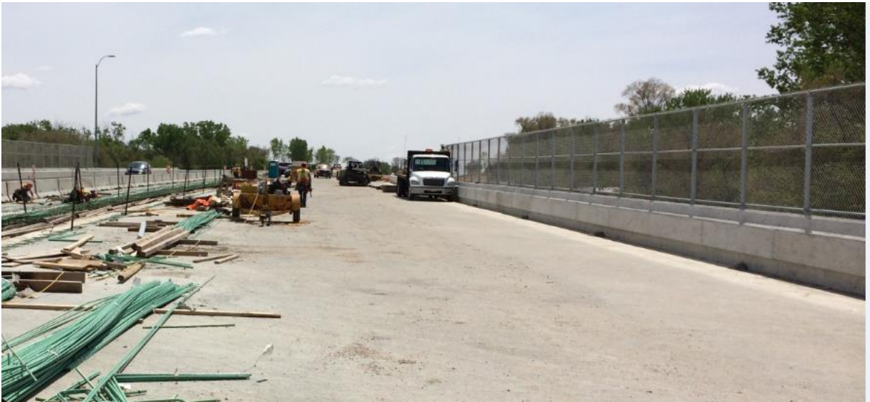
Figure 5.8 Completed Phase 2 with preparation for closure pour (May 14, 2014)
