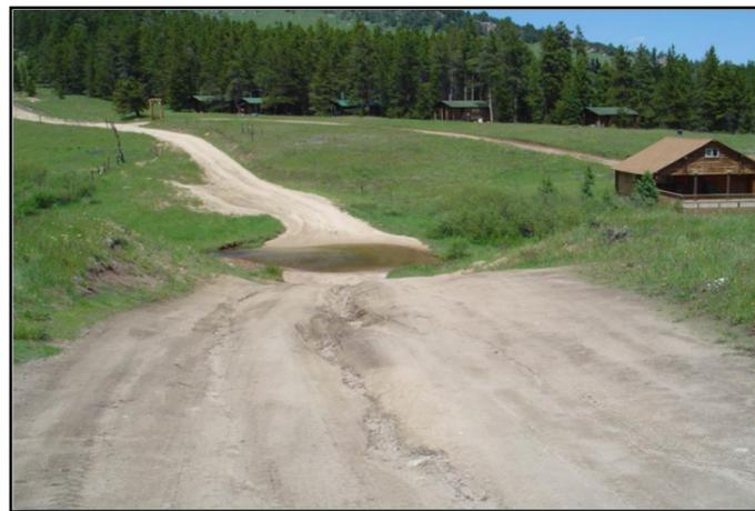
Figure 1.2 Loss of crown (WTTC, 2014)
