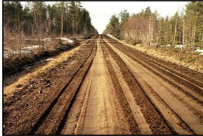
Figure 1.5 Severe rutting damage (ROADEX, 2014)
