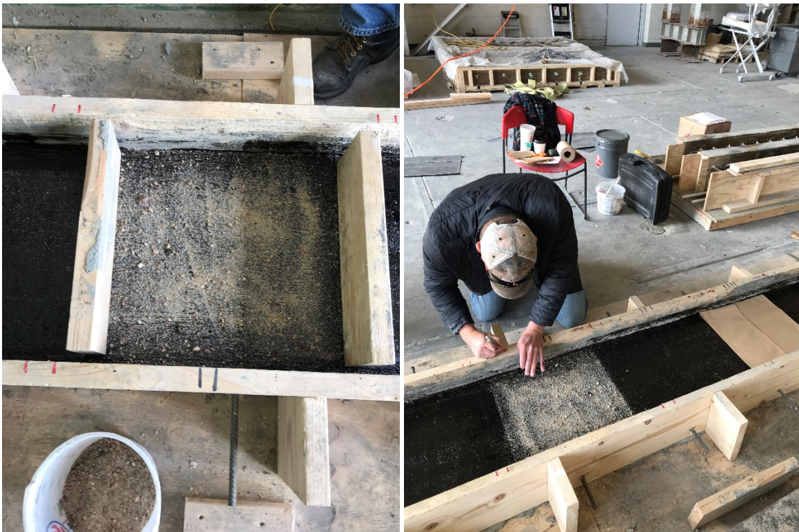
Figure 29. Segment B2: Placement of the gravel under the membrane
