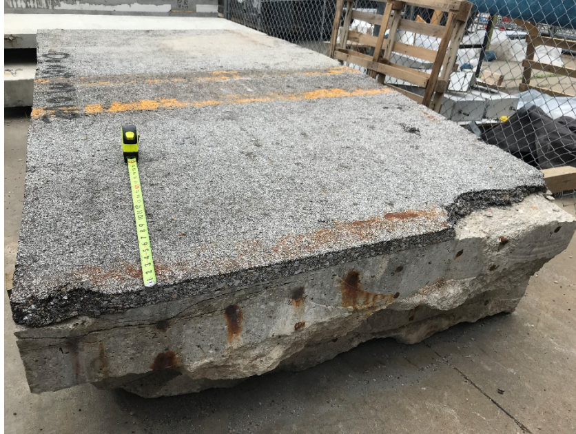
Figure 42. Field Specimen. View from North End showing the nine rebars
