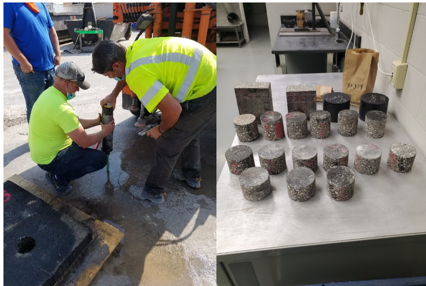
Figure 10. Coring (left) and all density test specimens (right)
