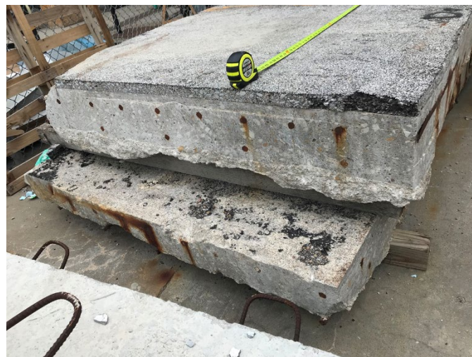
Figure 45. Field Specimen. View from South End showing the nine rebars
