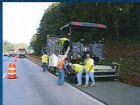
New Concrete Placed
