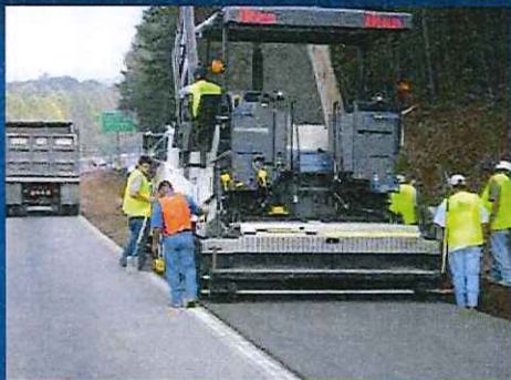
New Concrete Placed
