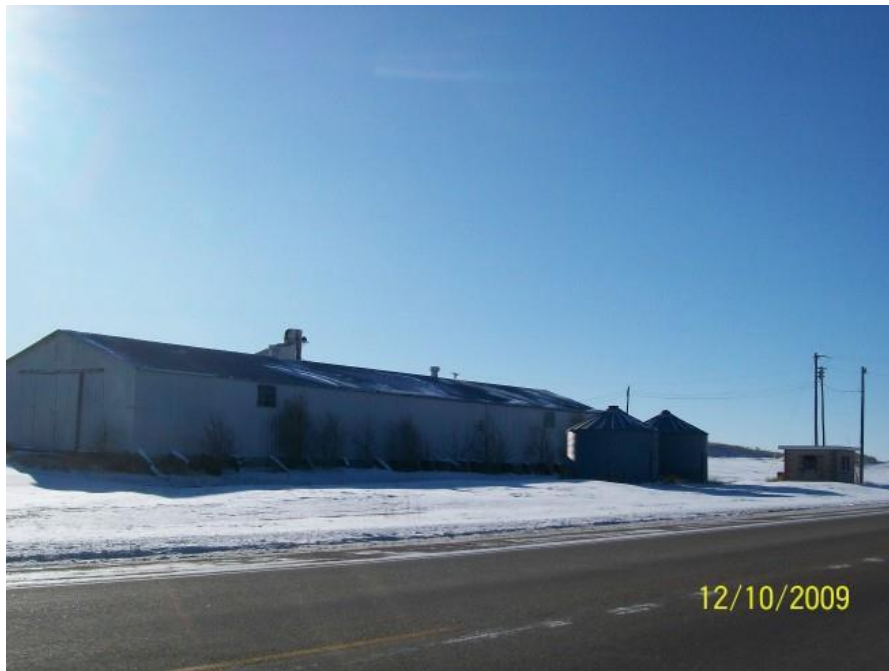
Figure 4. View of FN2015-02, steel storage bridge, steel grain bins and concrete block scale house. Morrill County Assessor photo.
