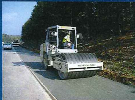
Roller Compaction (rubber-coated drum)
