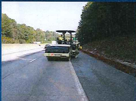
Initial Roller Compaction
