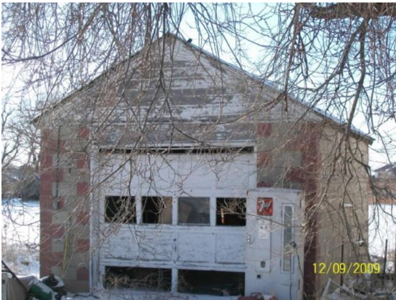
Figure 3. View of FN2015-01, garage. Morrill County Assessor photo.
