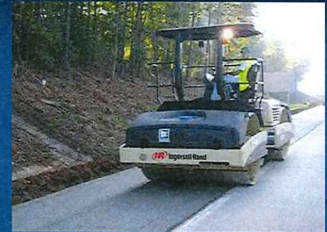
Initial Roller Compaction
