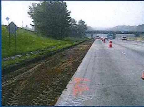
Base Ready for Compaction
