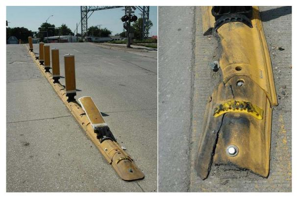
Figure 4.1. Flattened and abused curbing due to overrunning trucks in Waverly
