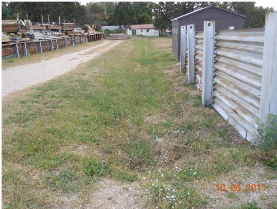
Figure B.4 Infiltration trench before construction
