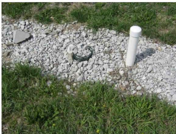
Figure 3.8 Upstream infiltration trench basket rock and observation well
