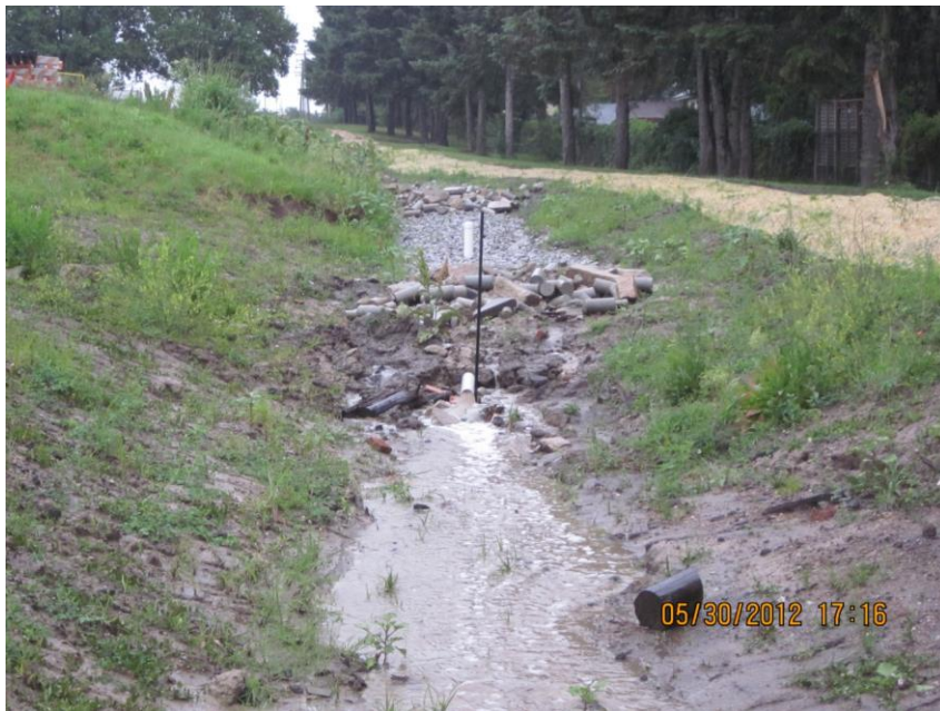
Figure B.13 Filter trench outlet during rain event
