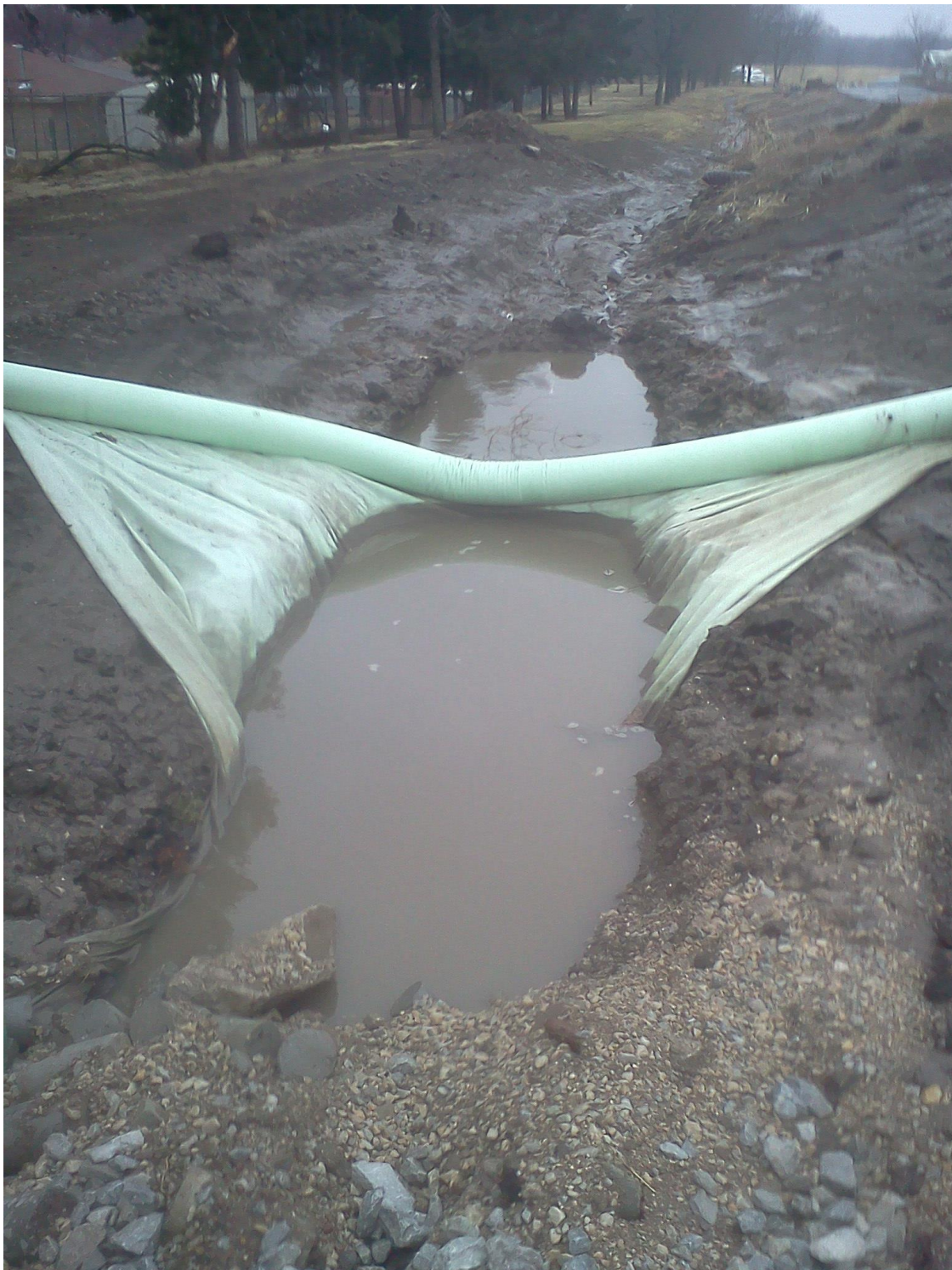
Figure B.12 Rain event during construction of filter trench
