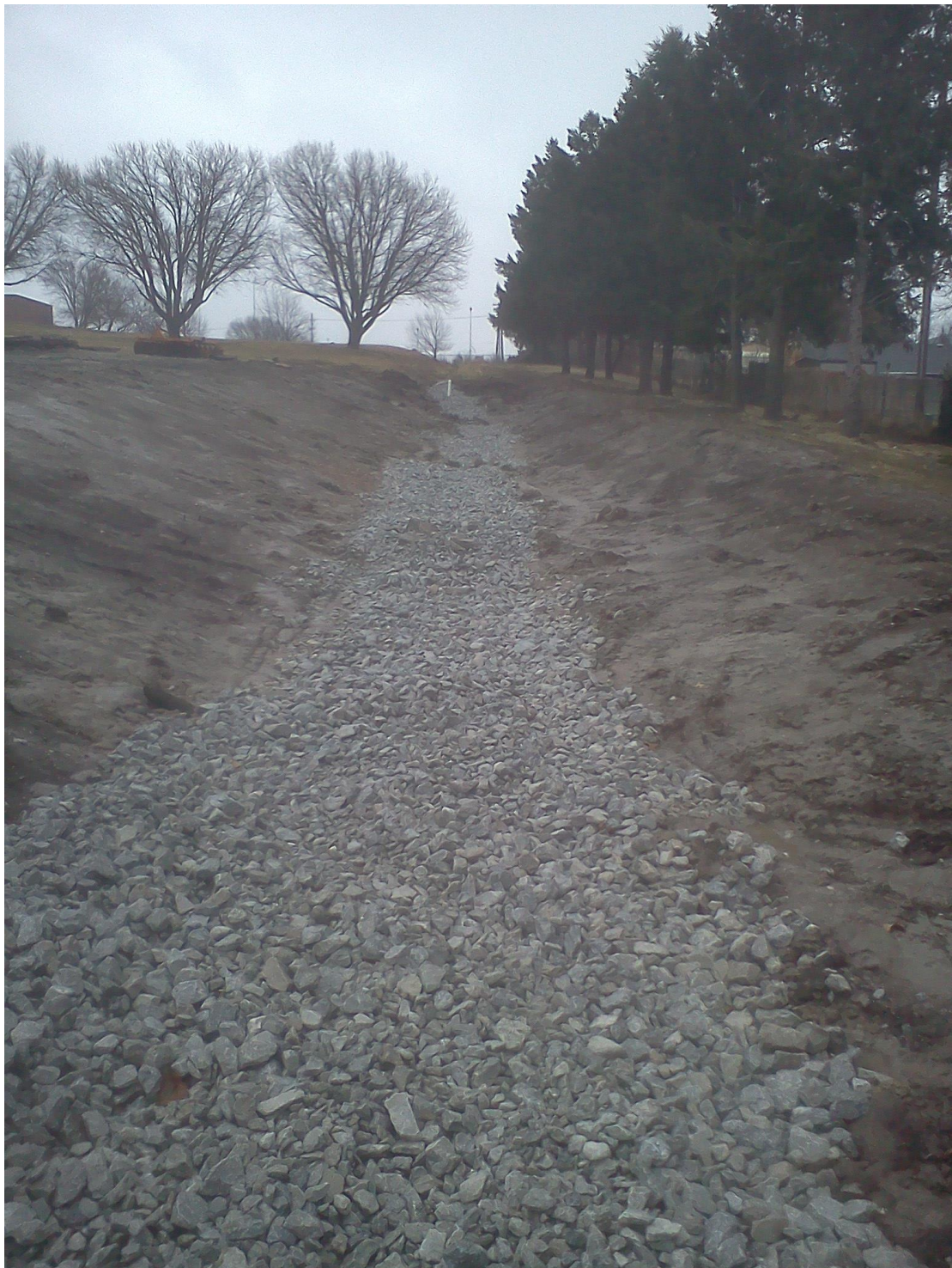
Figure B.7 Filter trench after construction
