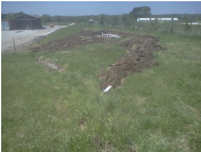
Figure B.8 Bioretention diversion during construction
