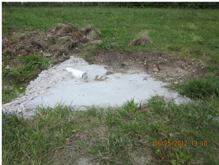
Figure B.9 Bioretention diversion after construction
