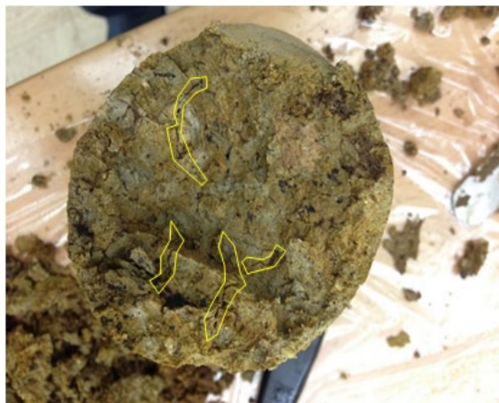
Figure 5.4 Cracks and fissures inside of the sample from IS-14.5 (I-180 and Superior St.)
