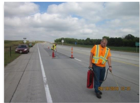
Figure 10 Sealer Application with Handheld Sprayers
