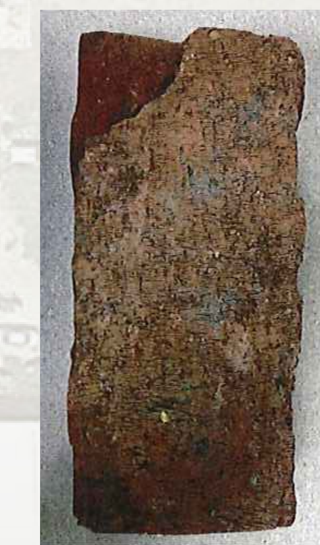
Damage on underside of bricks, not visible from surface
