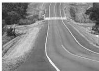
The portion of the roadway adjacent to the traveled way for accommodation of stopped vehicles, for emergency use, and for lateral support of the base and surface courses. On secondary roadways the shoulder usually consists of turf. On heavily traveled roads the shoulder is usually a bituminous mixture or concrete.
