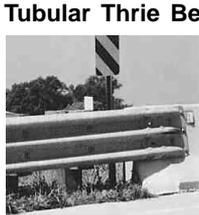
**Tubular Thrie Beam Retrofit Rail** Several of the bridges constructed years ago were provided with side rails that were designed to standards that have since been upgraded to better redirect errant vehicles. In front of the old rail a new metal beam retrofit rail is constructed, consisting of three corrugations similar to a guard rail, and will redirect most vehicles.
