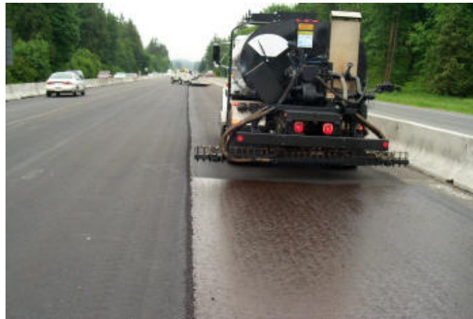
Figure 1-1. Typical tack coat applications.
