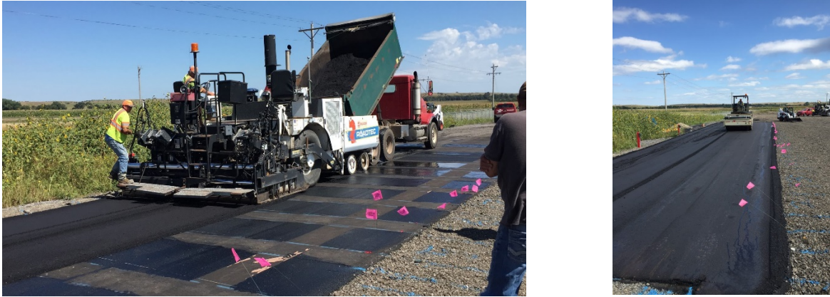
Figure 4-9. Paving the thin lift on the tack coated surface.
