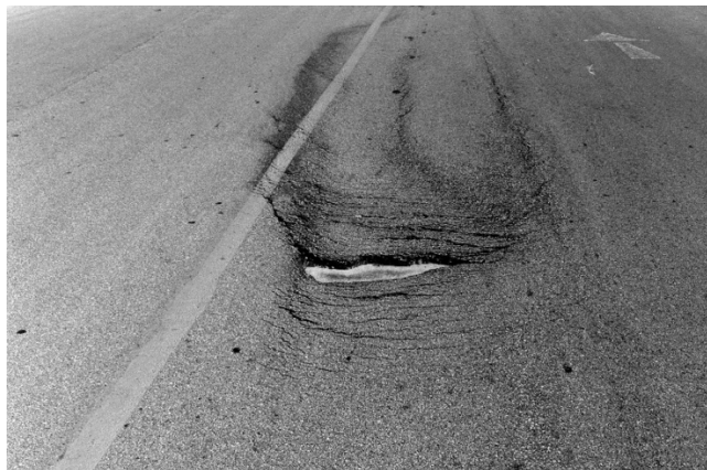
Figure 2-2. Slippage cracking.
