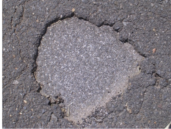
Figure 2-1. Delamination distress.
