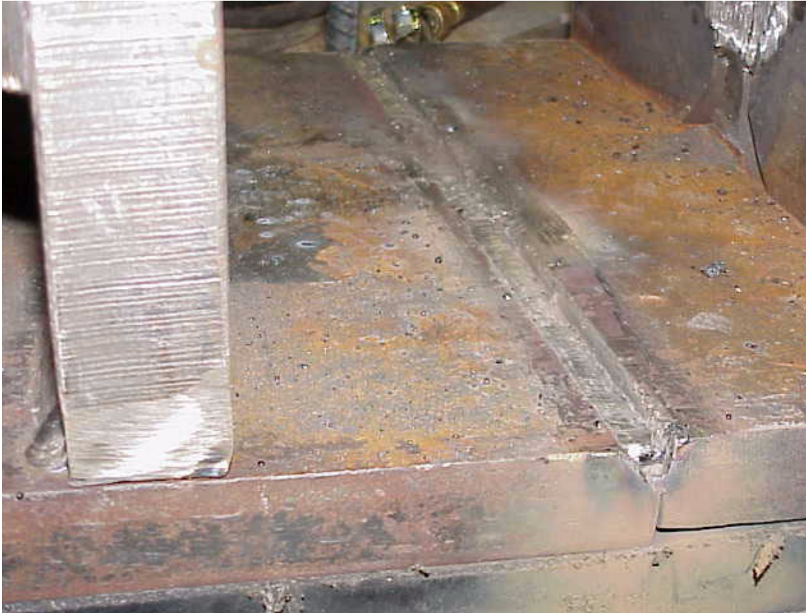
Figure 6-19: Bearing Pad After Welding
