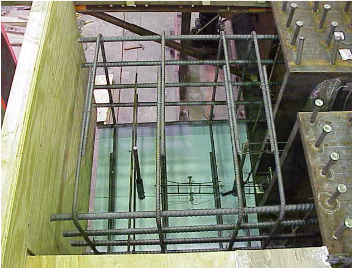
Figure 6-21: Diaphragm Reinforcing Layout
