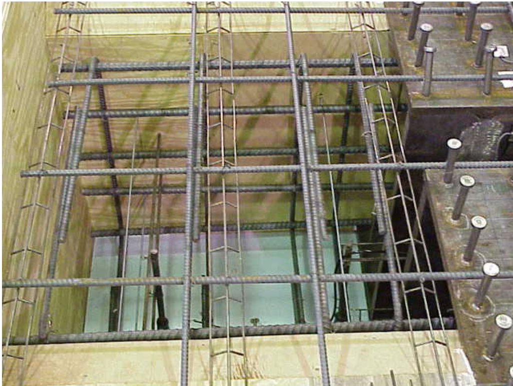
Figure 6-23: Completed Diaphragm Forming
