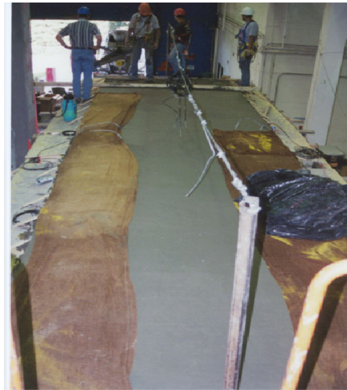
Figure 6-27: Casting of Deck Slab (Completed)
