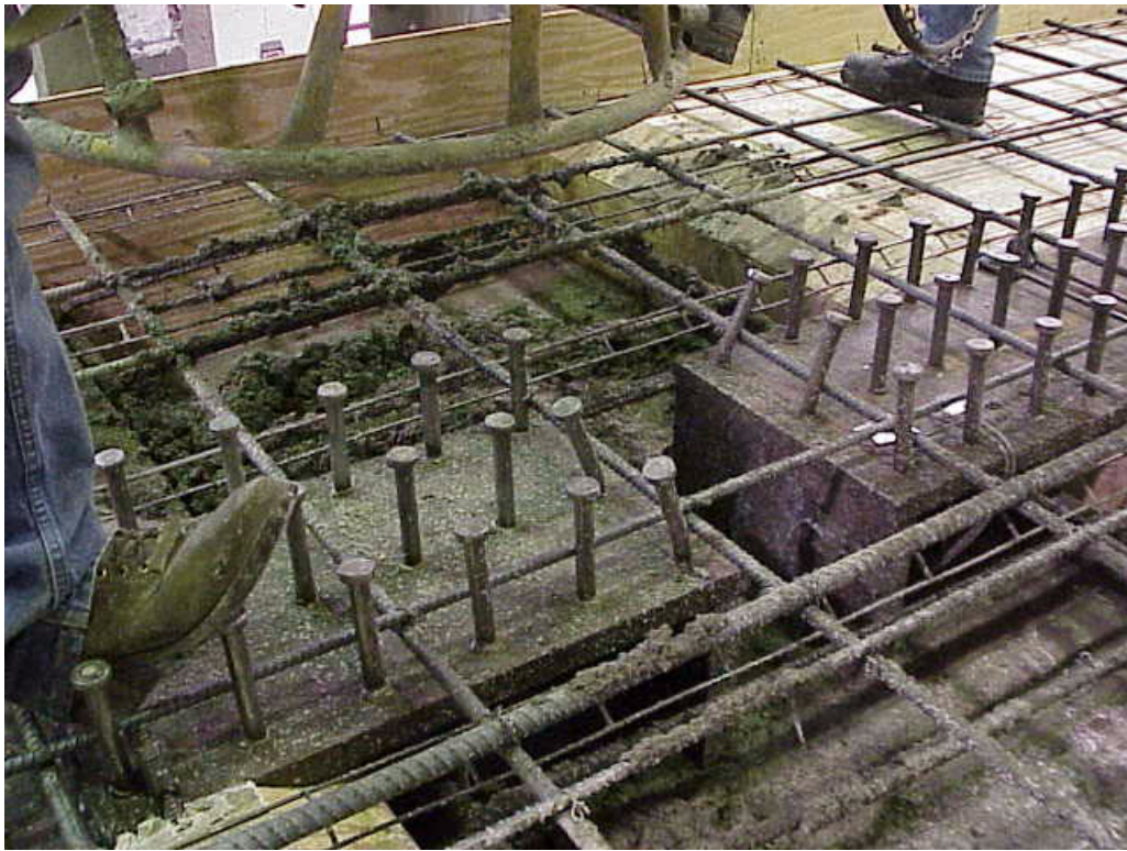
Figure 6-25: Completed Partial Diaphragm Casting
