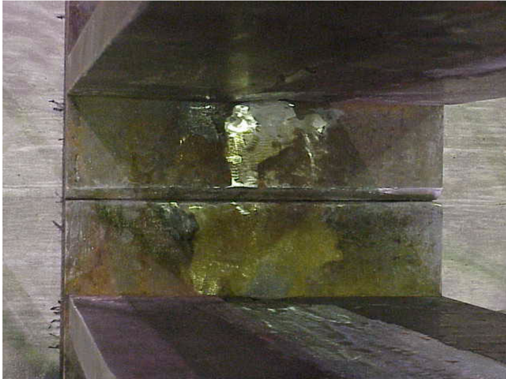
Figure 6-17: Girder Alignment Prior to Welding
