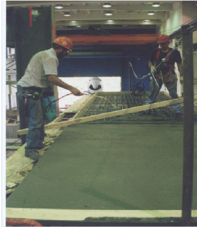
Figure 6-26: Casting of Deck Slab
