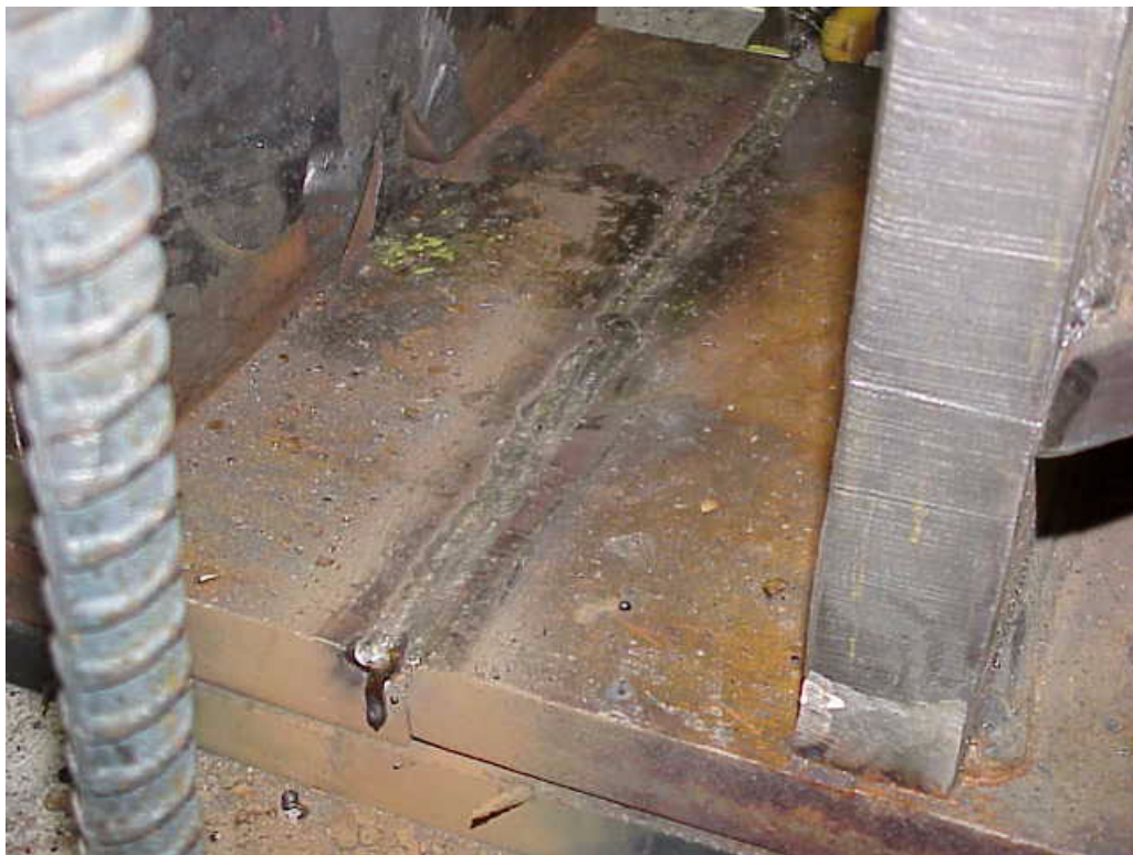
Figure 6-18: Flange Weld After Completion
