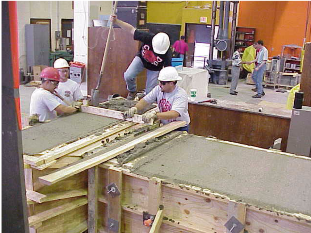
Figure 6-12: Casting of Pier Concrete
