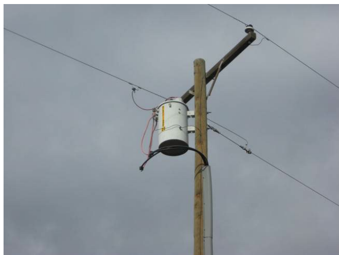
Pole-mounted electrical transformer in highway right-of-way.
