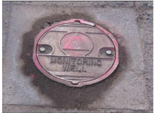
Typical in-ground monitoring well.
