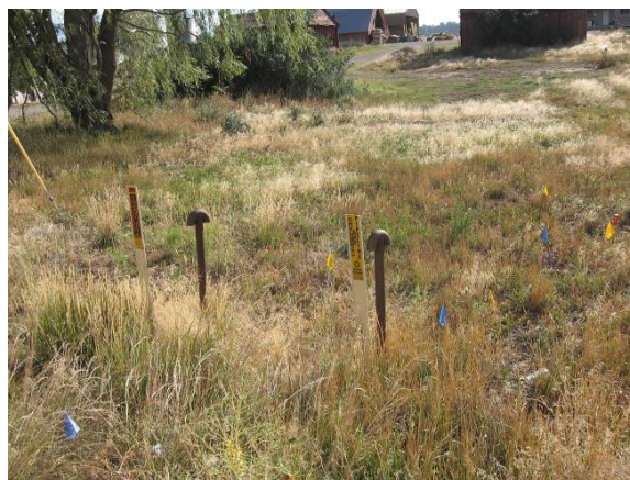
Gas pipeline vent pipes adjacent to highway right-of-way.
