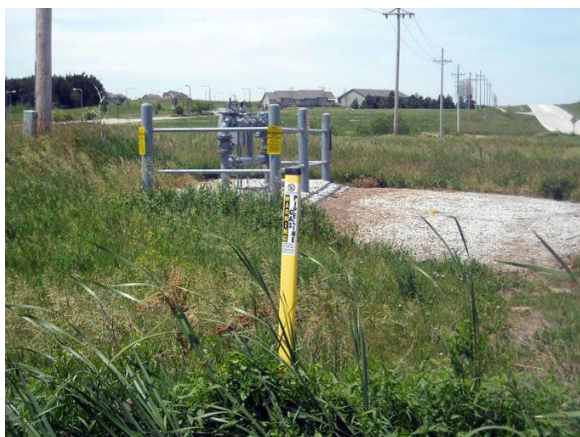
Gas line marker and regulator (background).
