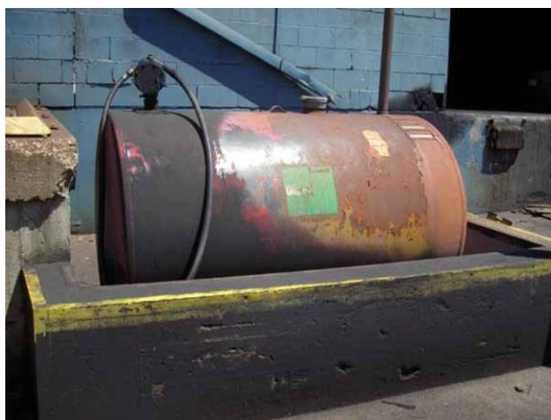
Typical used oil AST, with secondary containment in a concrete structure.
