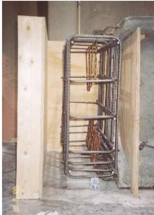
Figure 4.7 Elevation of Reinforcement in the End Block (B3E2)
