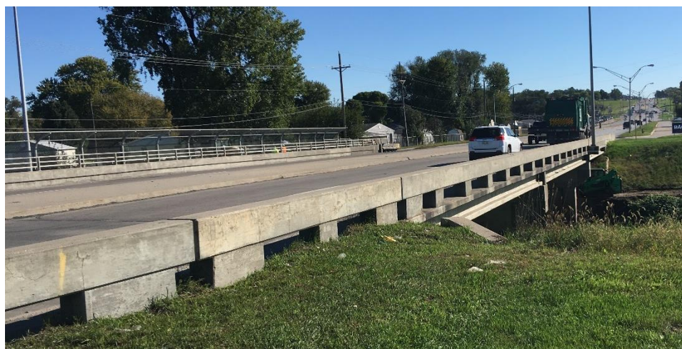
Figure A.85: Photo of bridge S275 18587.
