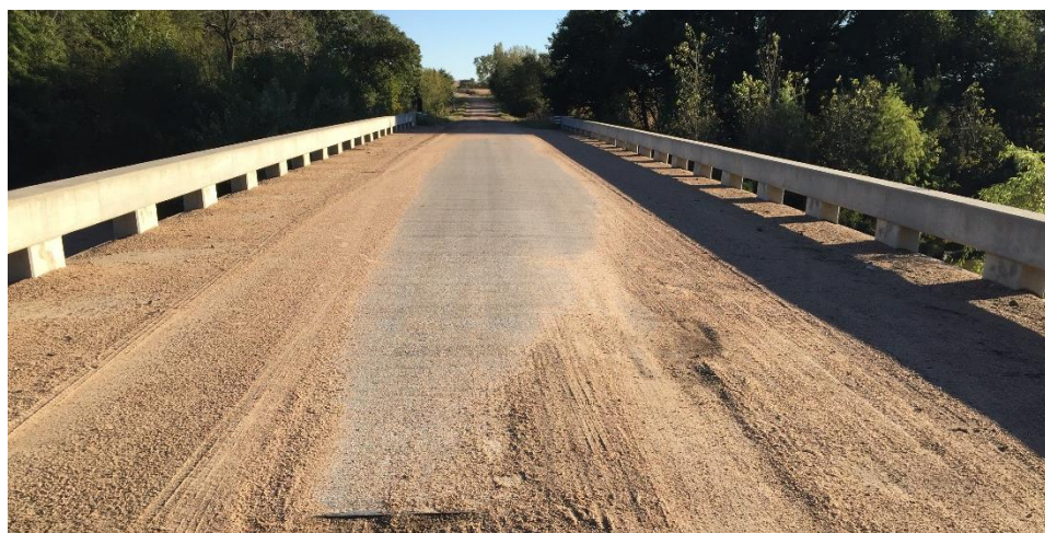
Figure A.99: Photo of bridge C008504145.
