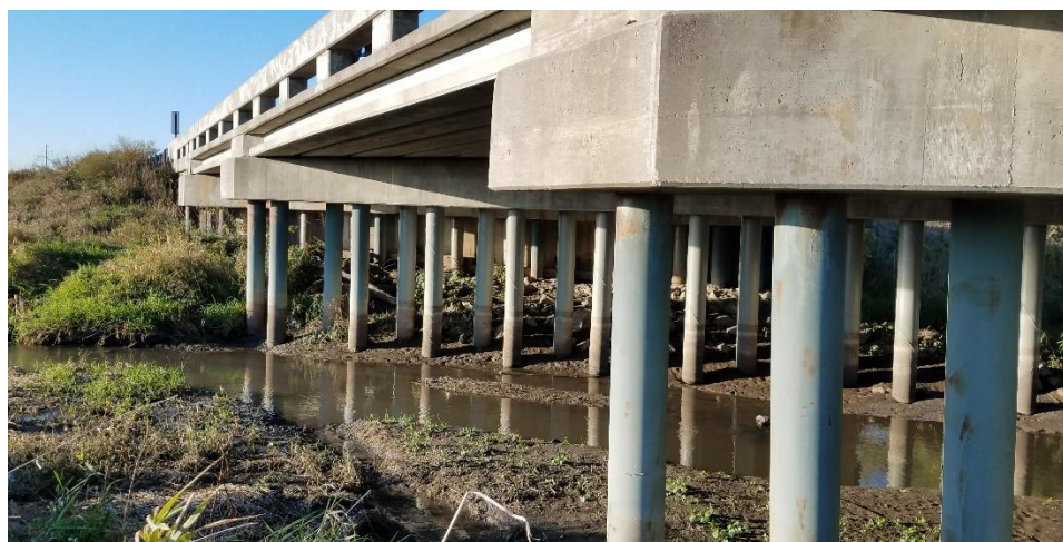
Figure A.21: Photo of bridge S009 00888.
