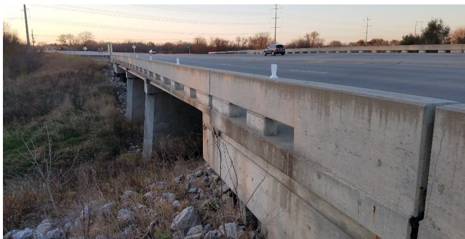
Figure A.30: Photo of bridge S034 31644.
