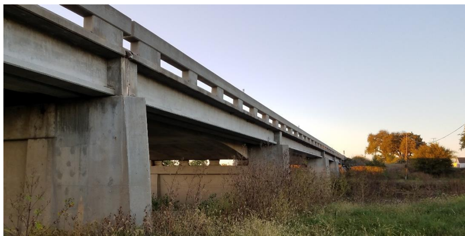
Figure A.78: Photo of bridge S103 02465.
