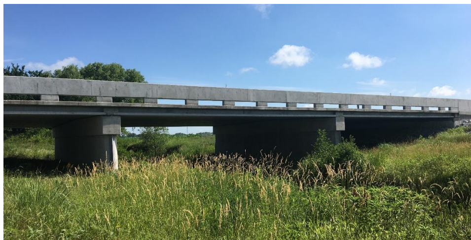
Figure C.77: Photo of bridge S080 40927R.
