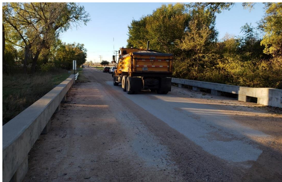
Figure 6.5: Photo of load case I for bridge C002408505.
