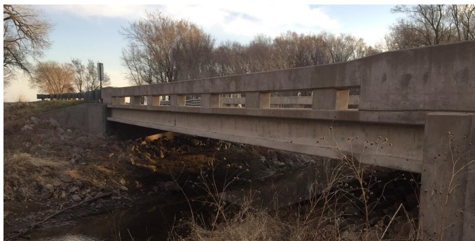
Figure A.93: Photo of bridge C002408505.
