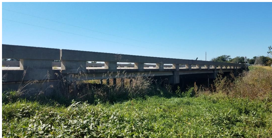
Figure A.2: Photo of bridge S006 26001.
