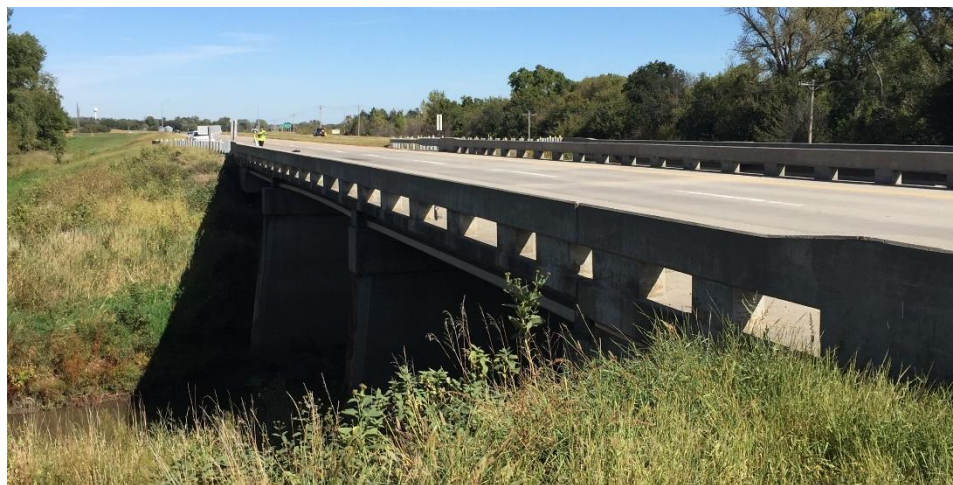
Figure C.86: Photo of bridge S081 05152L.
