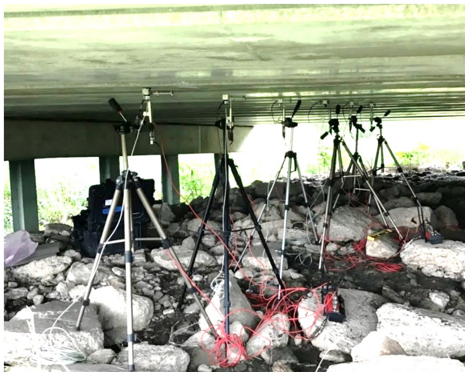
Figure 6.1: LVDT and strain gauge setup for bridge S006 26001.
