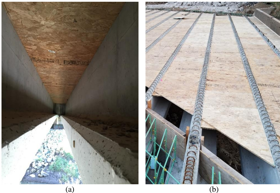
Figure 2.4: Stay-in-place plywood forms spanning between girders.
