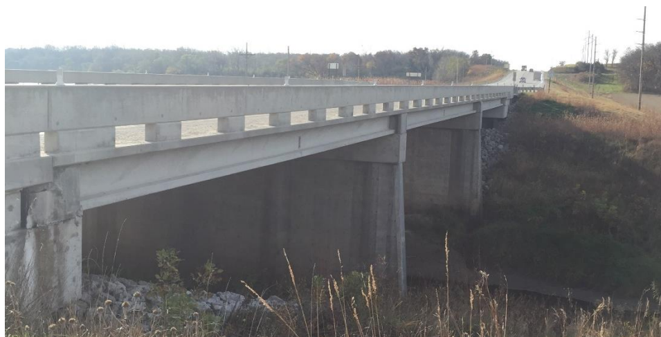
Figure A.42: Photo of bridge S050 06686.
