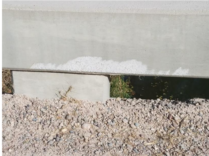
Figure A.107: Concrete patched rail on bridge M011022220.
