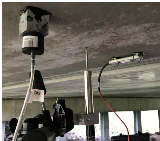
Figure 6.2: Accelerometer, LVDT, and strain gauge installation for bridge S006 26001.
