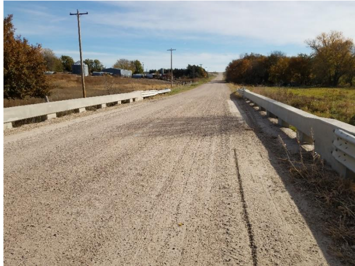
Figure A.105: Gravel covered deck on bridge M011022220.
