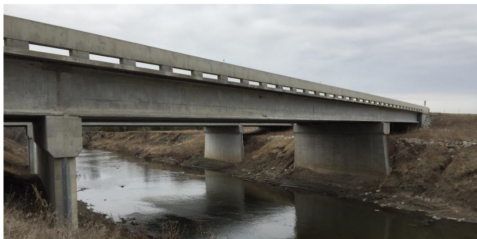
Figure C.52: Photo of bridge S080 40797R.
