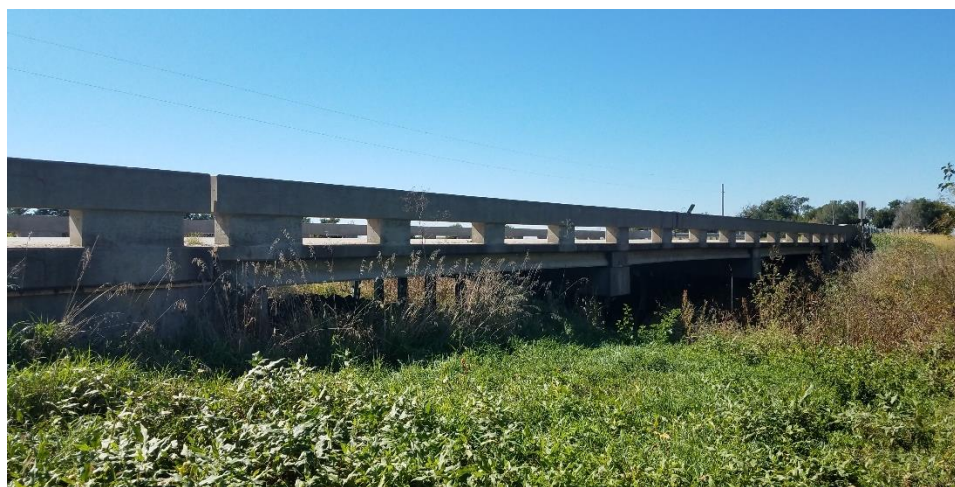
Figure C.2: Photo of bridge S006 26001.
