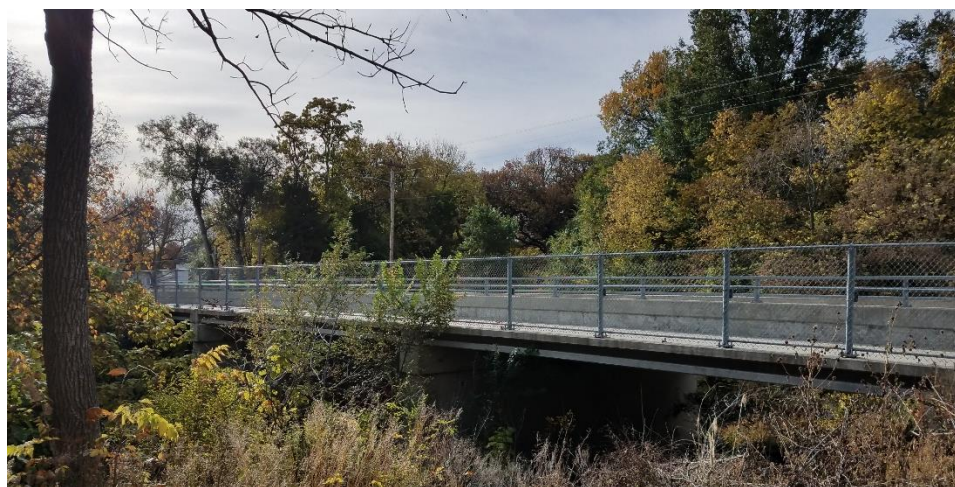
Figure C.34: Photo of bridge S058 00994.
