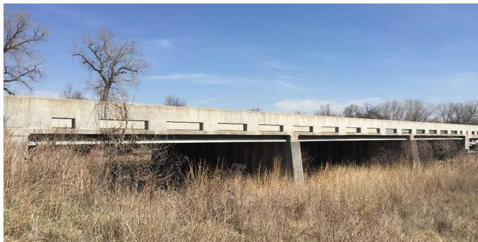
Figure C.95: Photo of bridge S089 06047.
