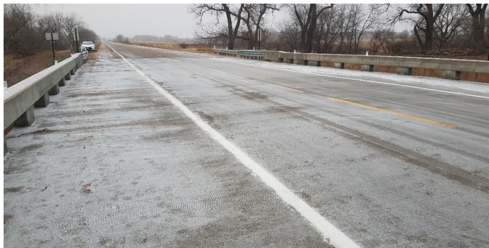
Figure C.27: Photo of bridge S020 32260.
