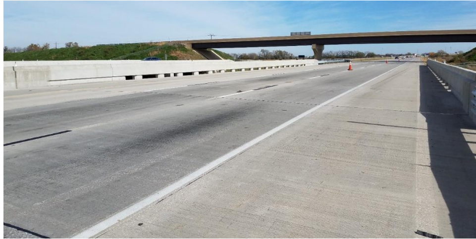
Figure 4.3: Photo of bridge S080 40872R.
