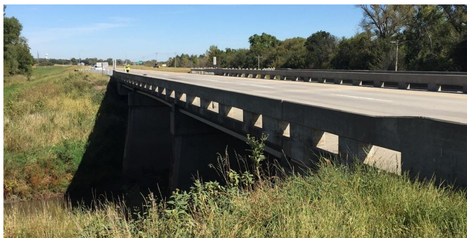
Figure A.67: Photo of bridge S081 05152L.
