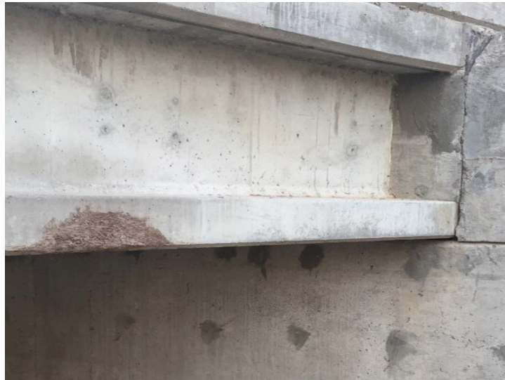
Figure A.96: Concrete patches on bridge C002408505.
