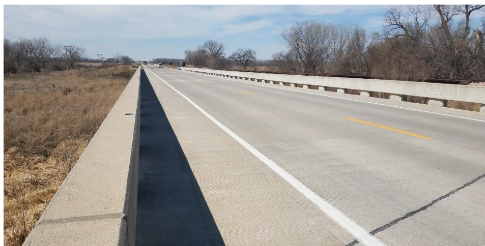
Figure A.75: Photo of bridge S089 06062.
