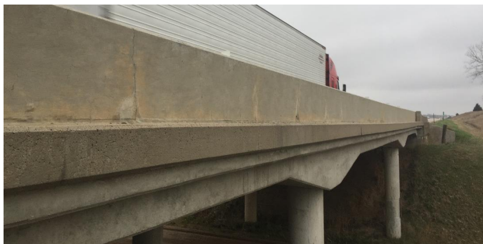
Figure C.43: Photo of bridge S080 38614R.
