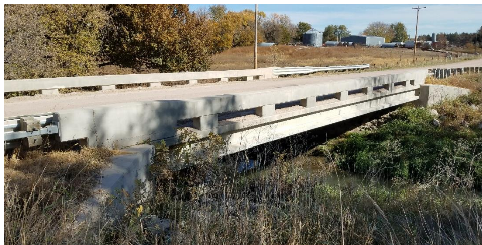
Figure A.104: Photo of bridge M011022220.
