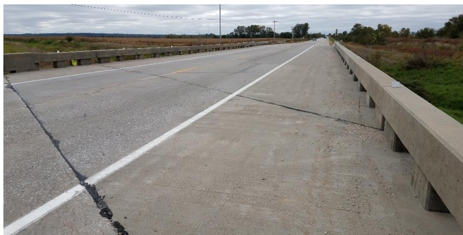
Figure A.10: Photo of bridge S006 34277.
