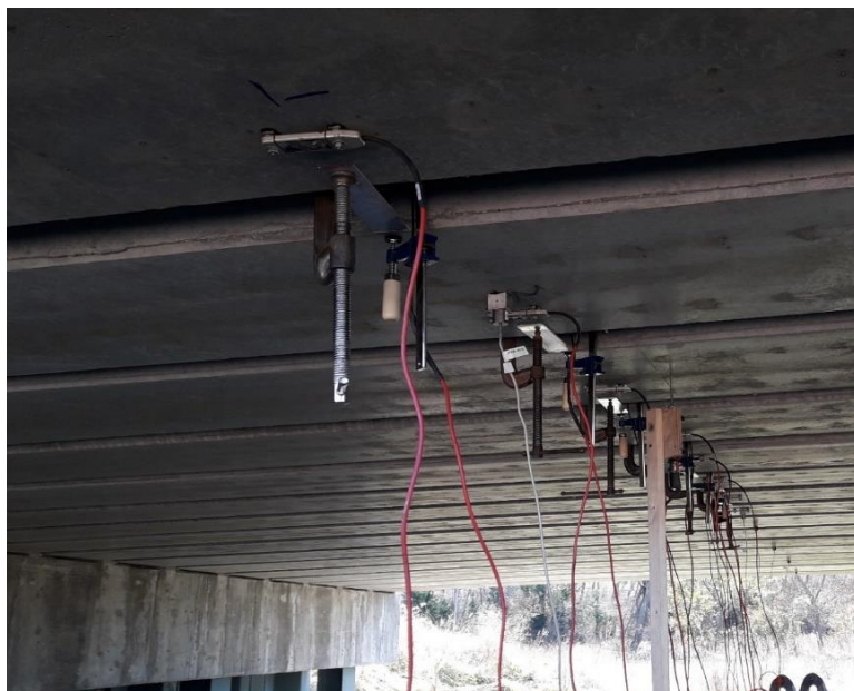
Figure F.15: LVDT and strain gauge setup for bridge S089 06047.
