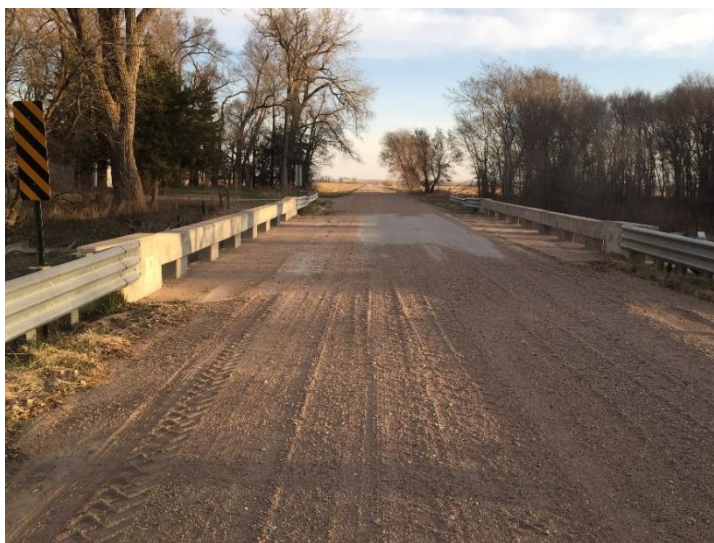
Figure A.94: Gravel covered deck on bridge C002408505.
