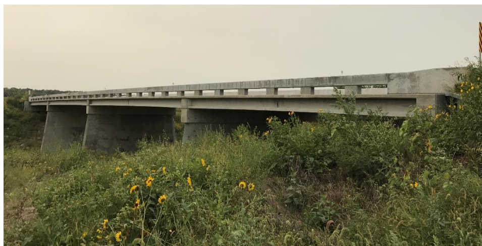
Figure A.109: Photo of bridge C004931110.
