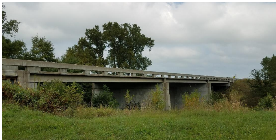
Figure A.37: Photo of bridge S050 04149.
