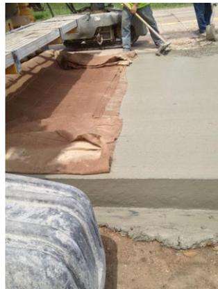
Figure 6. Placement of 40%RCA-60% 47B Fine
