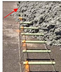
The red arrow shown is the dowel bar translation movement during concrete placement. Figure 1.
