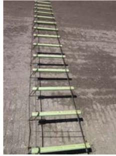
Figure 6. Uncut Tie Wires Dowel Bar Assembly
