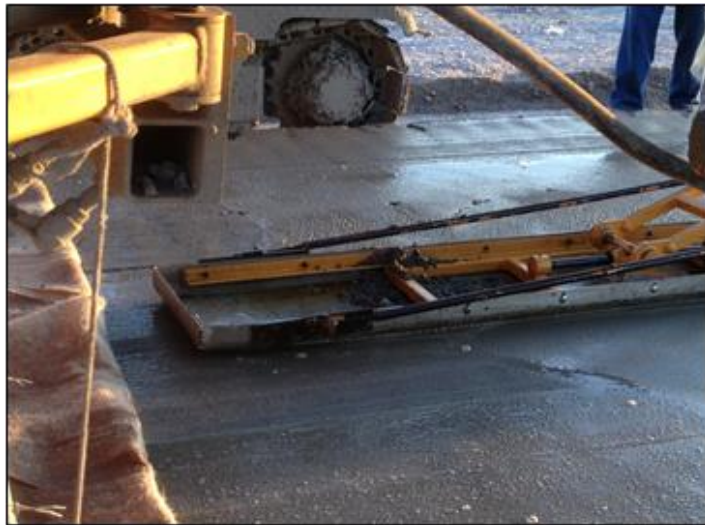
Figure 2. Placement of BX Concrete with Class B Aggregate
