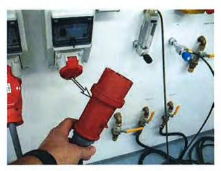
Figure 8.2: Disconnect the mains power
