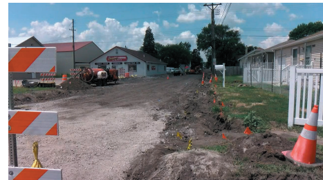
Figure 6: Photo at Michigan Ave. and 7th St. During Reconstruction.
