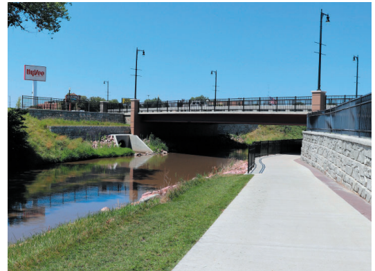
Figure 2: Photograph of underpass path reconstruction on Norfolk Avenue and 1st St. Credit to City of Norfolk Engineering Department
