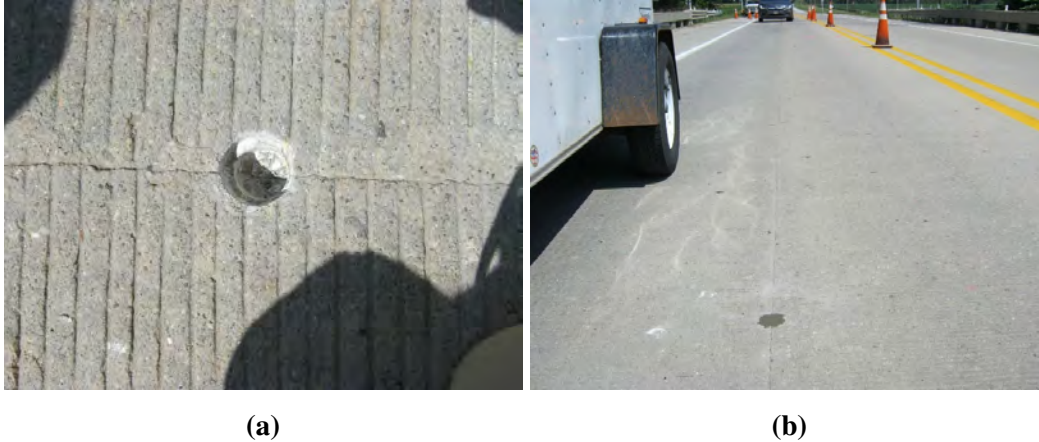
Fig. 4.2. Photographs of a hole made for chloride sampling (a) and the patched hole (b) after sampling was complete.
