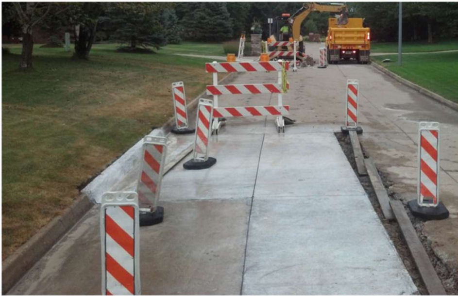
Concrete Patch (typically overnight)
