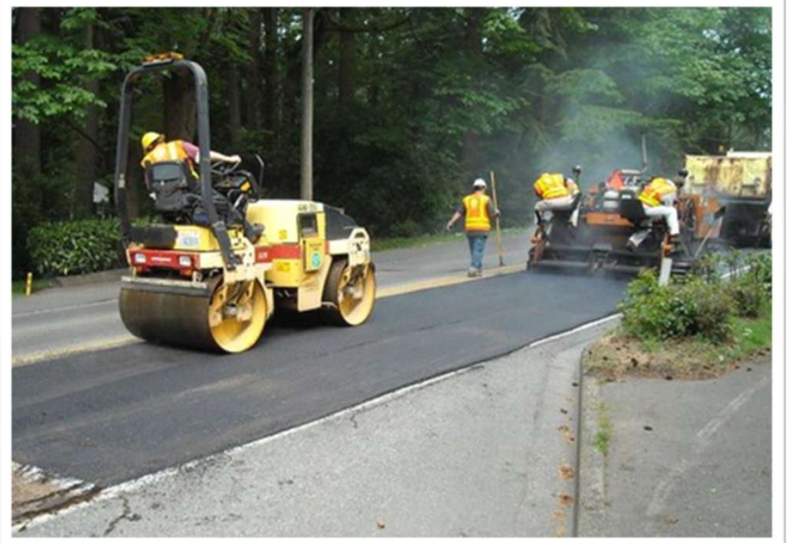
Asphalt Patch (one daylight period)
