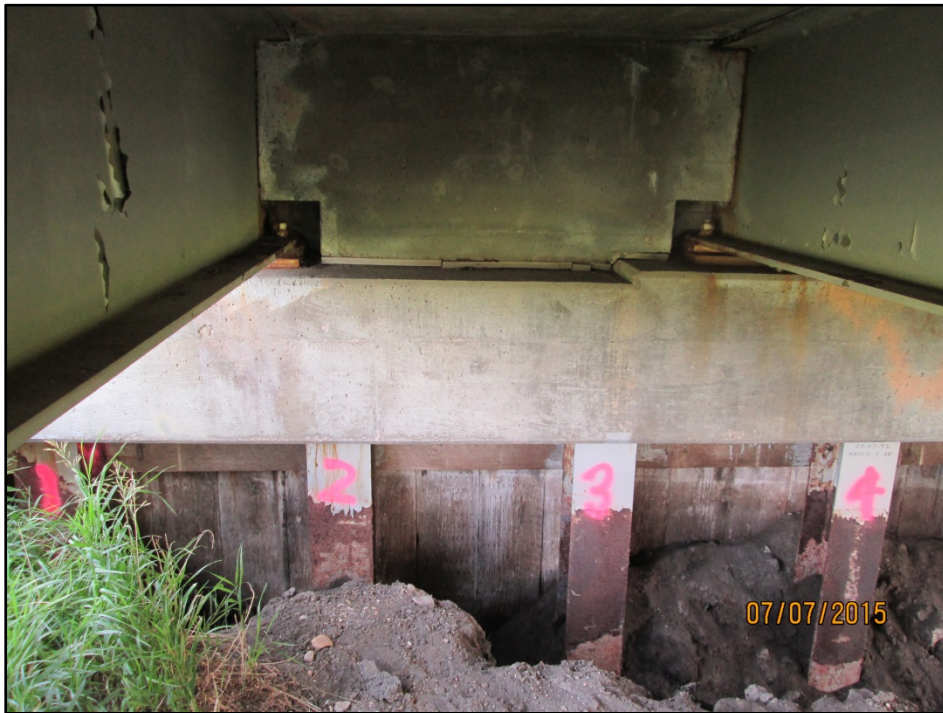
Photo 4: View of side of the structure. Orientation: East
