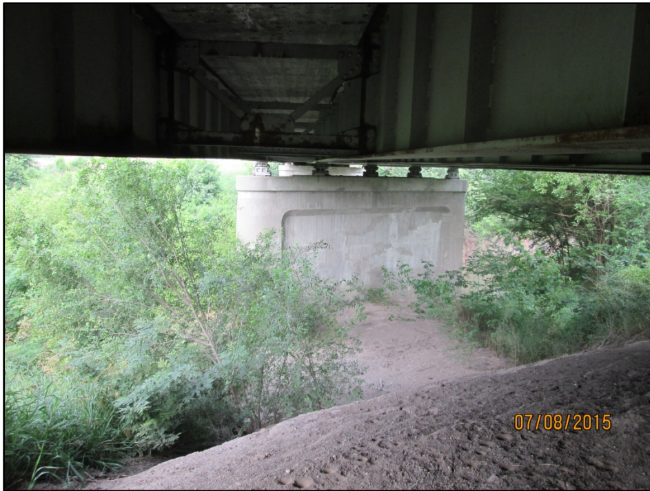
Photo 5: Midsection underneath bridge Orientation: West
