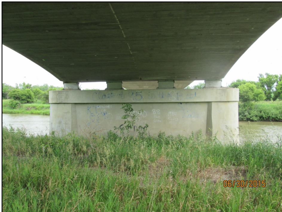
Photo 2: Side of structure under the bridge. Orientation: East
