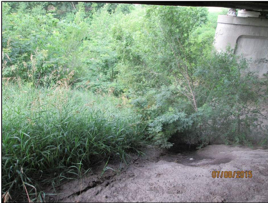
Photo 7: Area surrounding bridge structure Orientation: West
