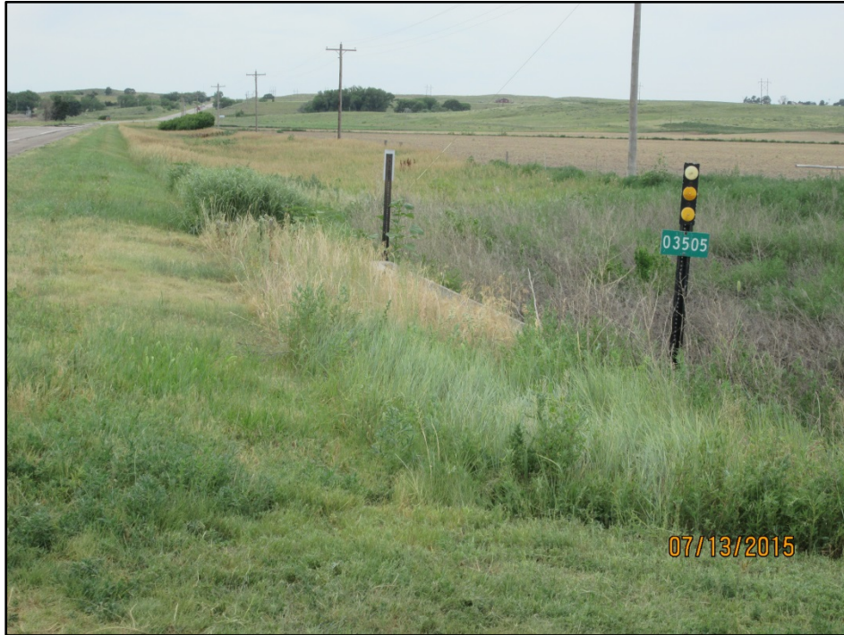
Photo 1: View along the side of the roadway. Orientation: West
