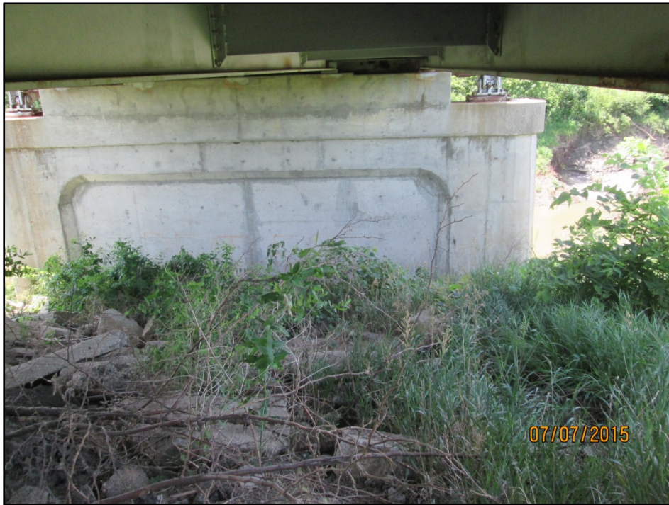
Photo 3: Underneath the structure. Orientation: West
