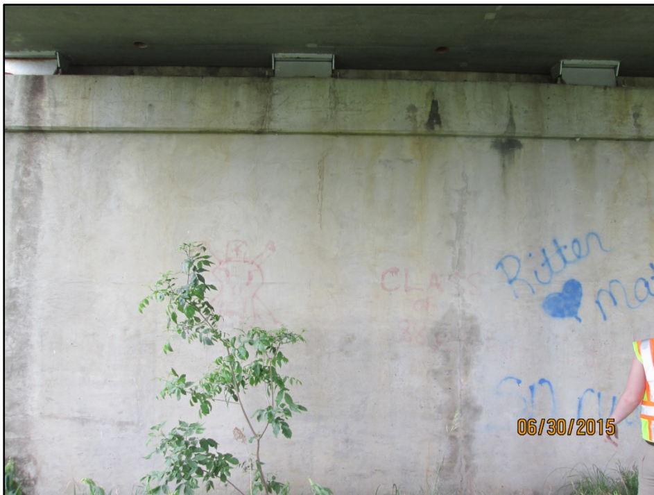
Photo 3: Side of structure. Orientation: West
