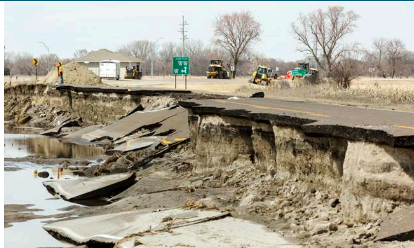
Left - The US-281 bridge over the Niobrara River was washed out when Spencer Dam collapsed.
