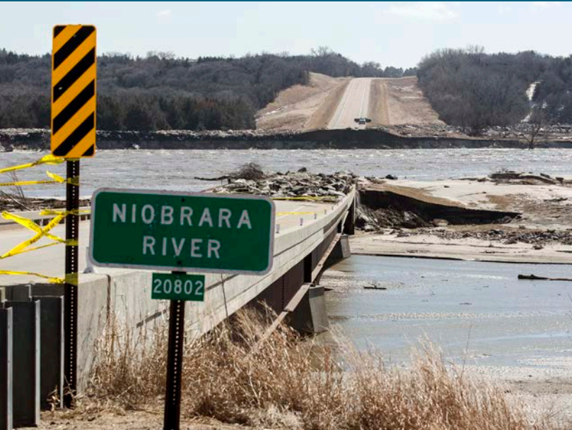
Left - The US-281 bridge over the Niobrara River was washed out when Spencer Dam collapsed.
