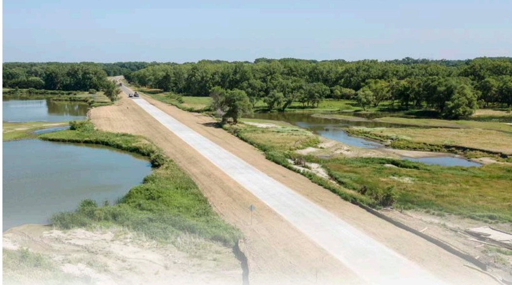
Reconstruction of Highway 39 at the Loup River overflow south of Genoa.
