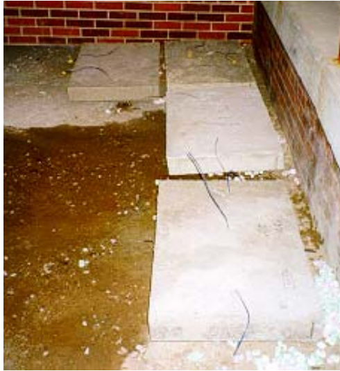
Figure 3-15(b) 3 ft x 2ft x 3.5 in. slabs
