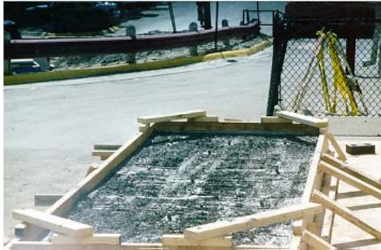
Figure 5-1(b) 6-in. conventional concrete layer
