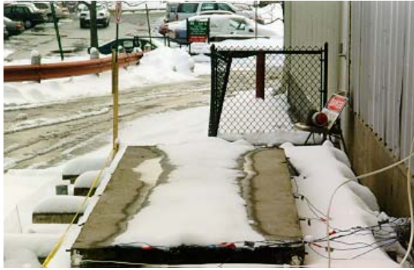
(b) Slab during testing
