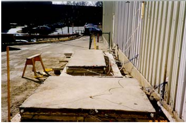
Figure 5-11(b) Slabs connected to power source
