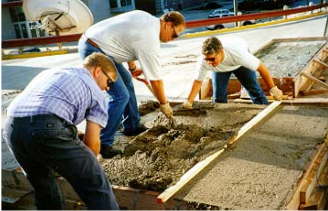
Figure 5-5 Conductive concrete mix showed excellent workability and surface finishability
