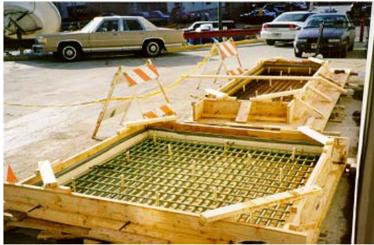
Figure 5-1(a) Slabs ready for casting the conventional concrete layer
