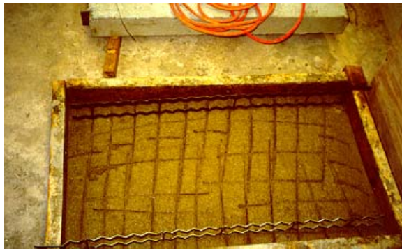
Figure 3-18 Sawdust layer was used as insulation layer
