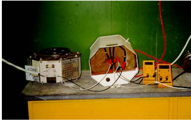
Figure 5-11(a) The VARIAC, Transformer and Amp-meters for Power Control
