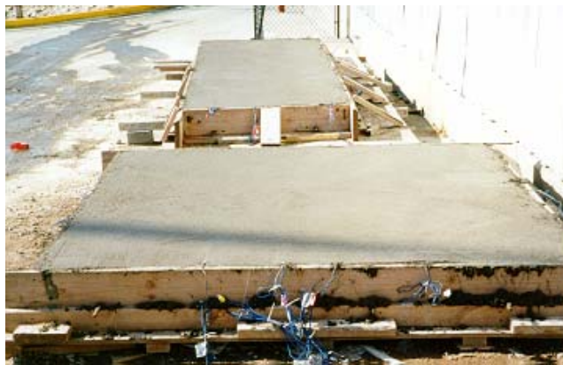
Figure 5-6 Slabs after finishing
