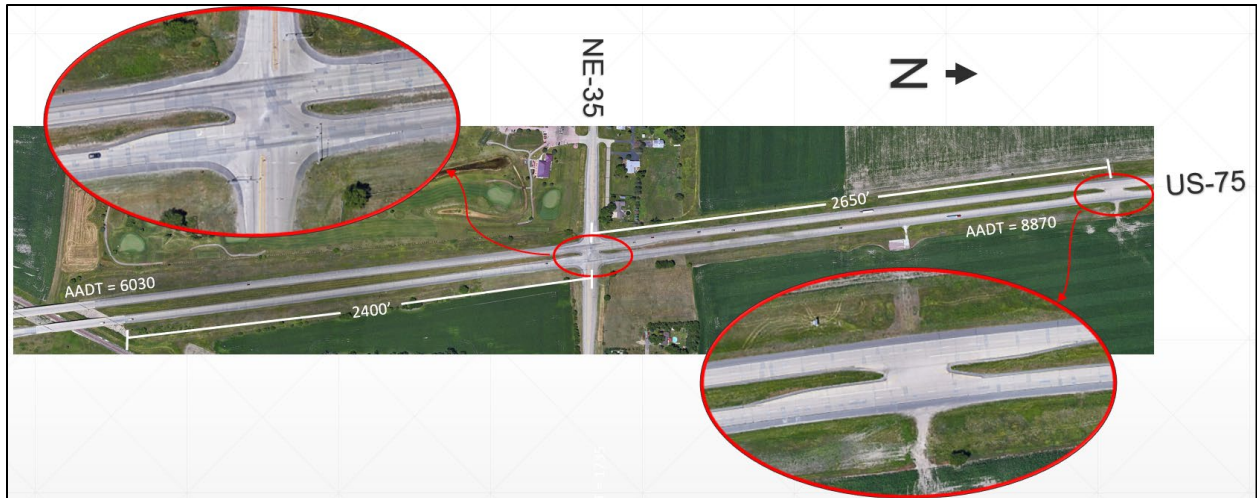
Figure 4.4 Intersection of US-75 and NE-35 near Dakota City, NE [22]
