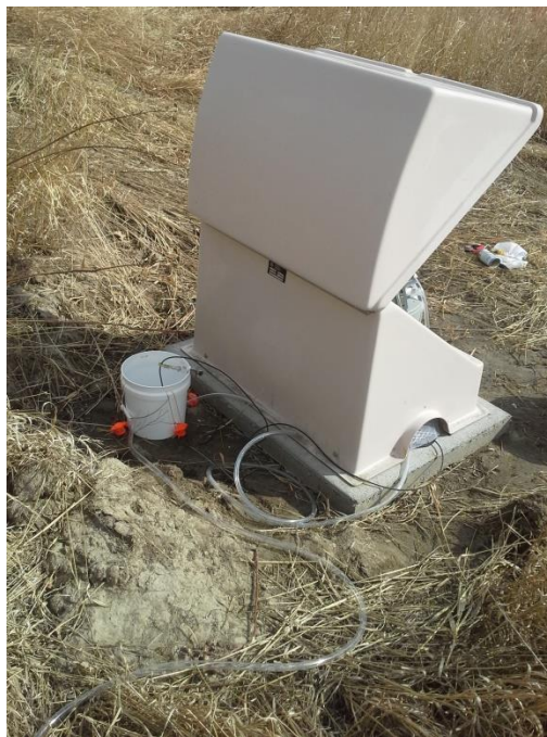
Figure 2.4 Bucket stacked near the security box at Highway 77 over Rock Creek
