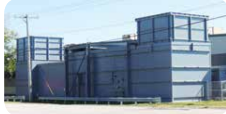
Duncan Aviation Engine Test Cell Building
