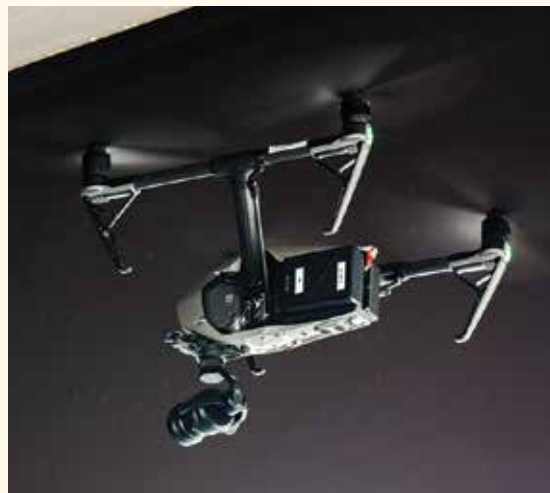
A drone hovers underneath a bridge in Omaha during inspections by NDOT bridge inspectors in June.
