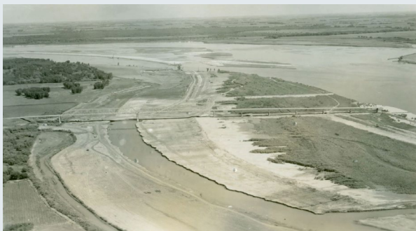
Photo: Partially completed bridge & USACE excavation, 1955.
