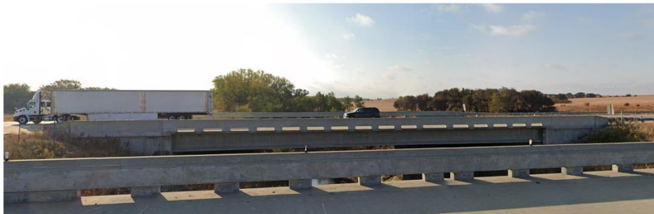
Prestressed concrete bridges (S080 41653 )
