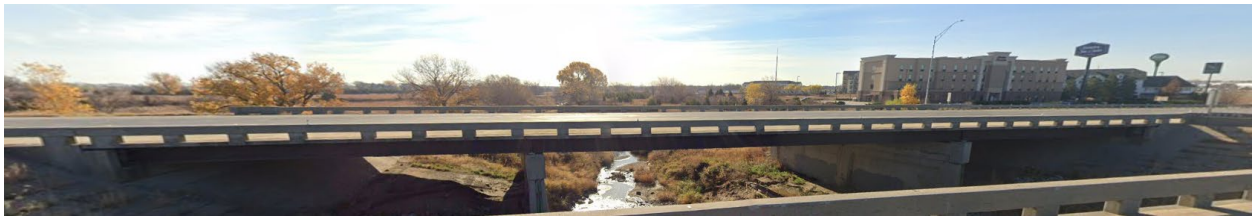
Figure 8.18 Steel Rolled Beam Three-Span Bridge (S080 40375) (Google Map, 2023)
