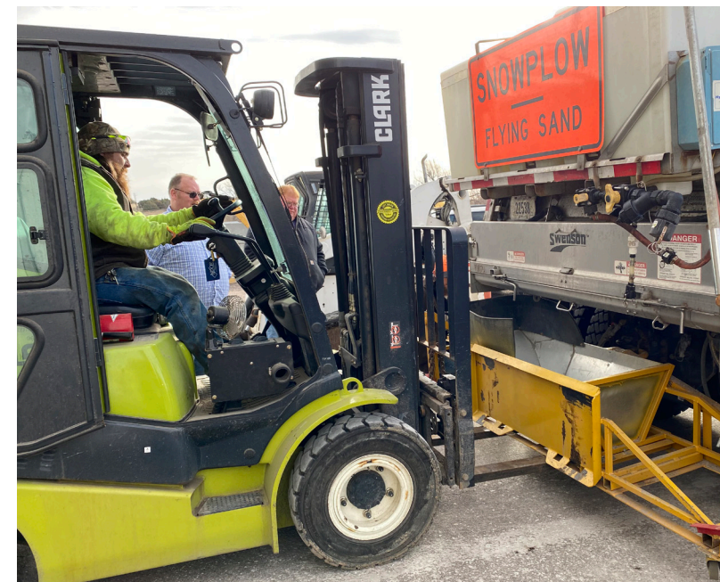
Maintenance operators remove the validation box to weigh salt collected.
