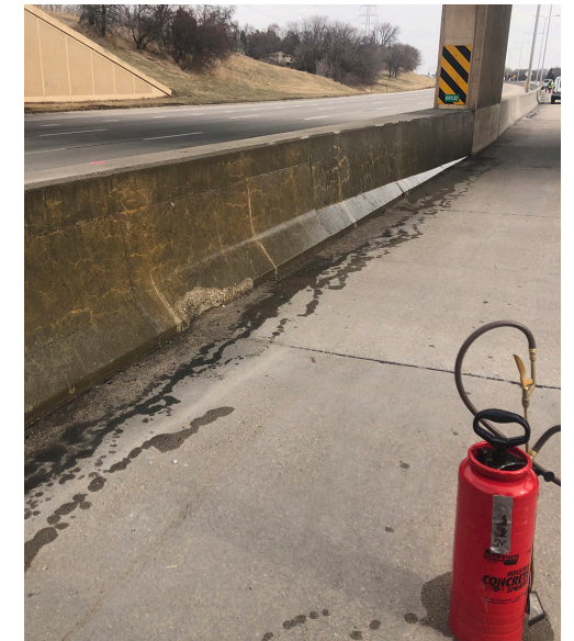
Pavement Design investigated the importance of power-washing vertical structures prior to reapplying penetrating concrete sealers.
