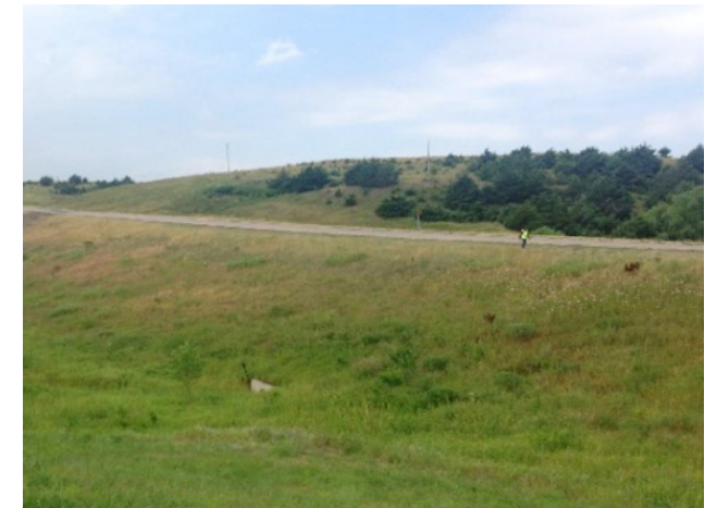
Verdigre slope at Highway 84
