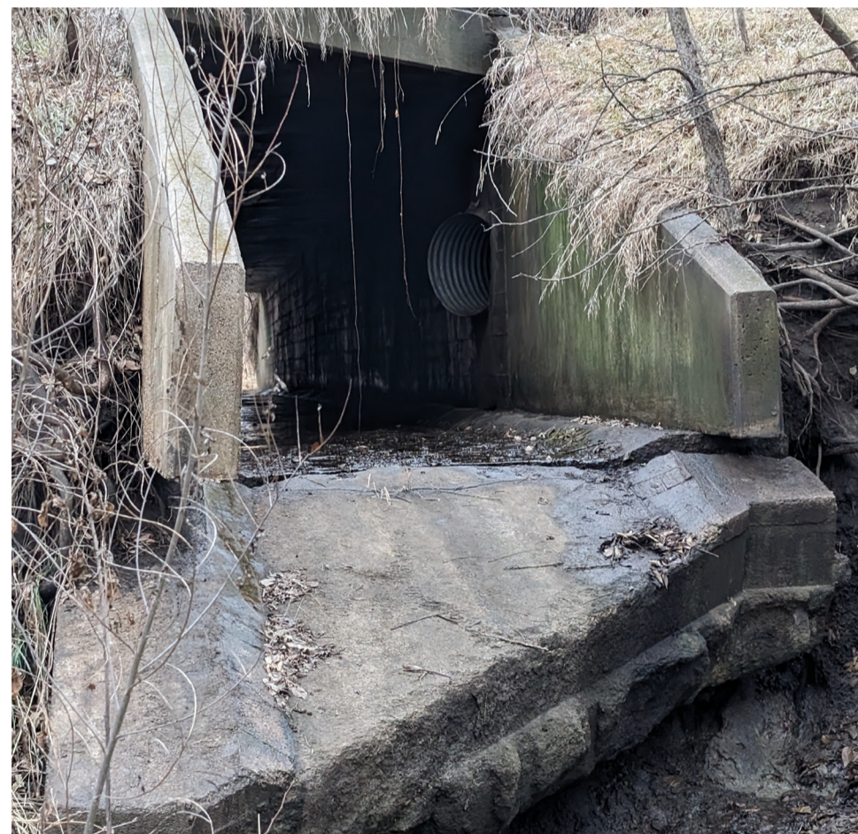
Degraded culvert outlet
