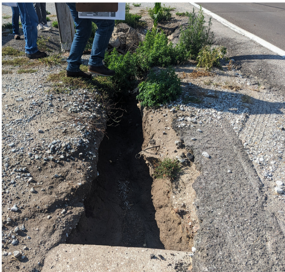
Erosion at edge of roadway
