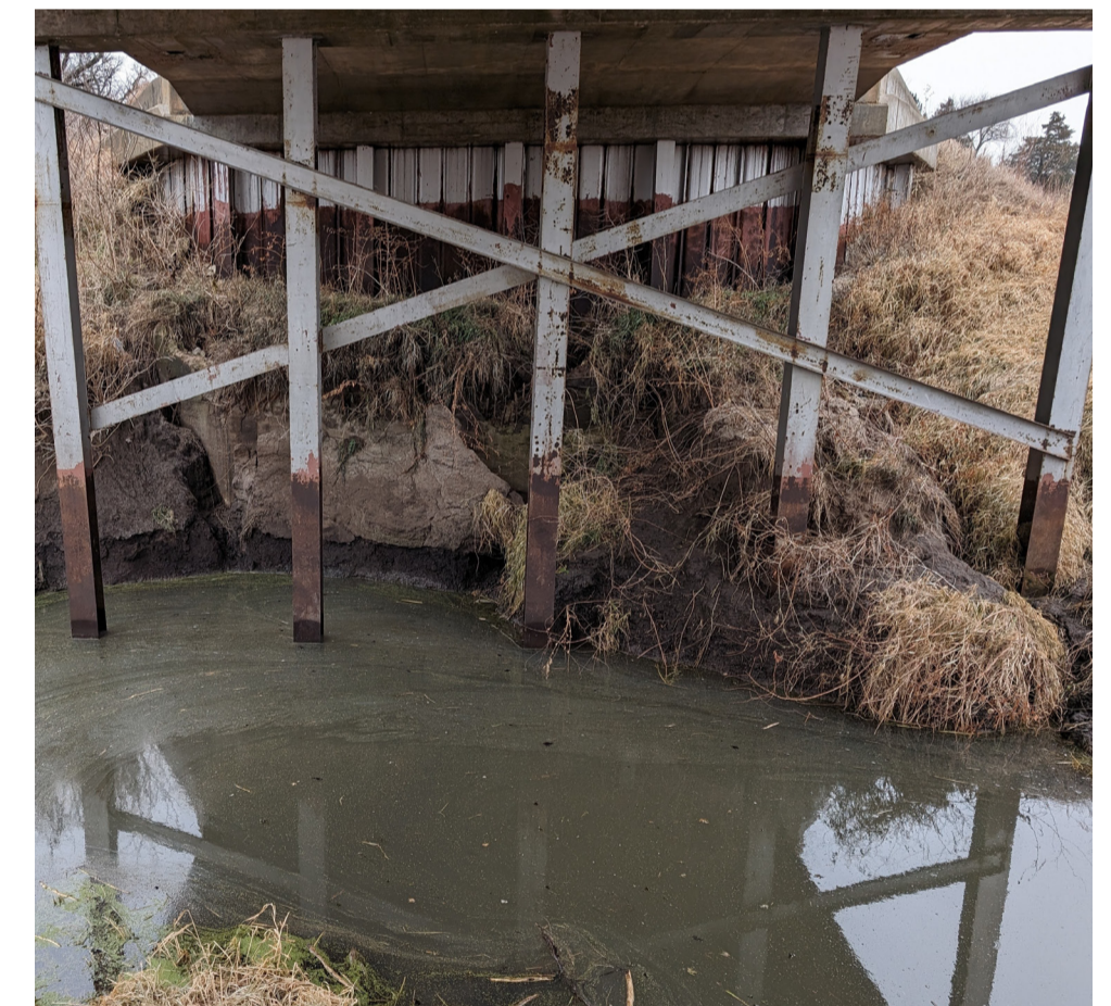
Scour and bank degradation near abutments
