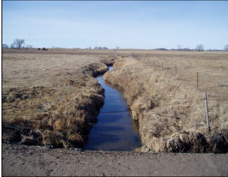
Item 327 Code: 9 EXCELLENT CONDITION Description: Channel perpendicular to roadway
