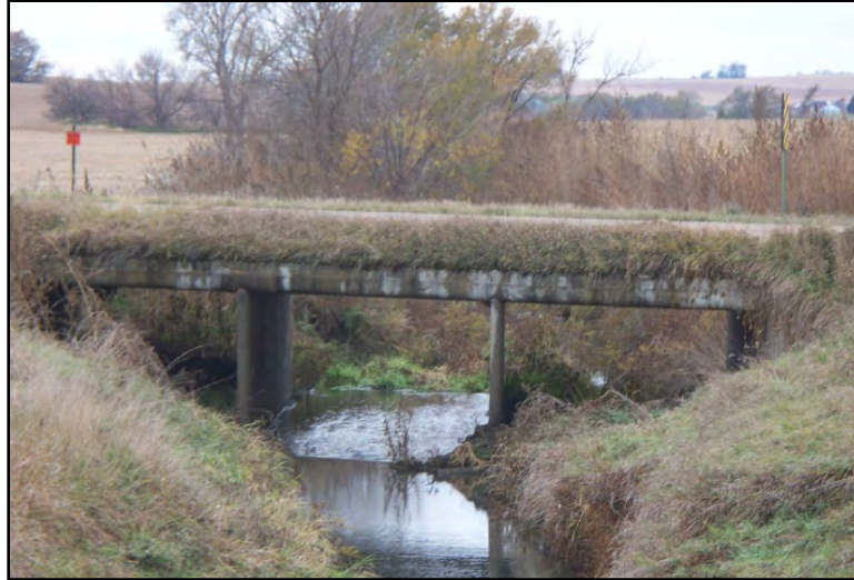
Item 335 Code: N Description: No major issues evident
