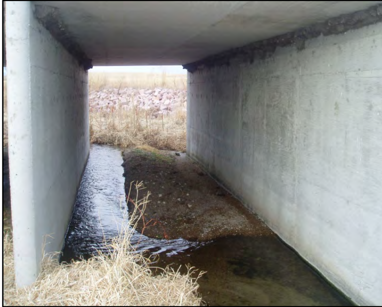
Item 323 Code: 9 EXCELLENT CONDITION Description: No deficiencies
