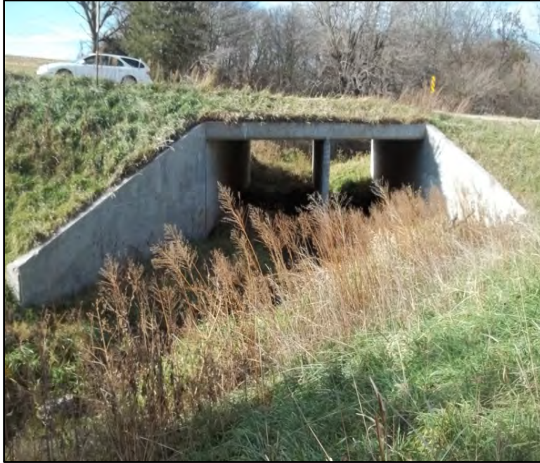
Item 324 Code: 9 EXCELLENT CONDITION Description: No deficiencies
