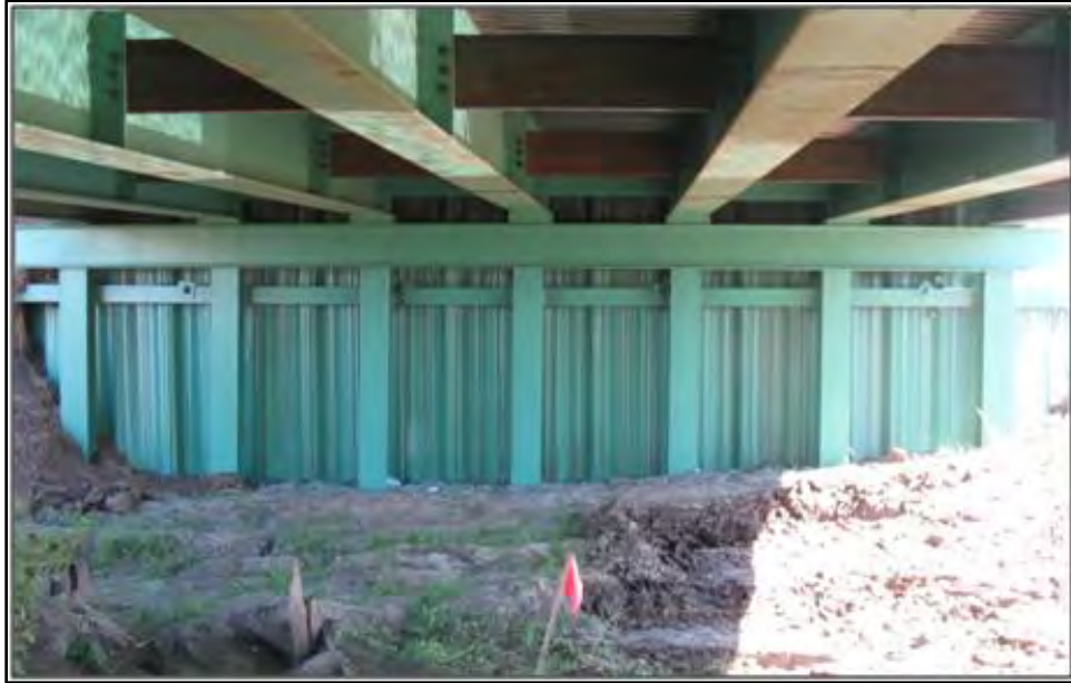
Item 311 Code: N not applicable Description: Steel plates here are shims, not a bearing device
