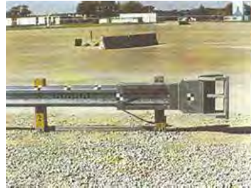
Beam Eating Steel Terminal
