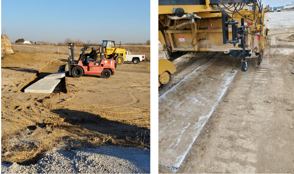
Figure 6.8 Milling process of concrete slabs using concrete deck milling equipment.
