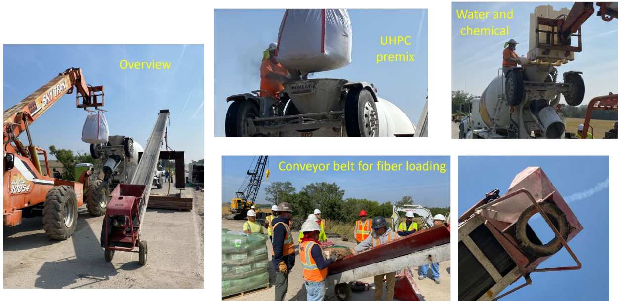
Figure C.4 IADOT Cass County Bridge Overlay Project – Batching.
