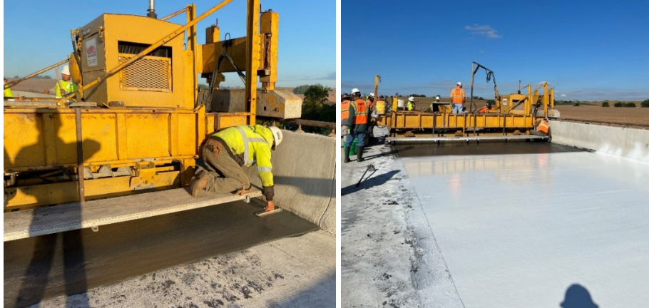
Figure C.8 From left to right: Hand-finishing after paving; Application of white curing compound.
