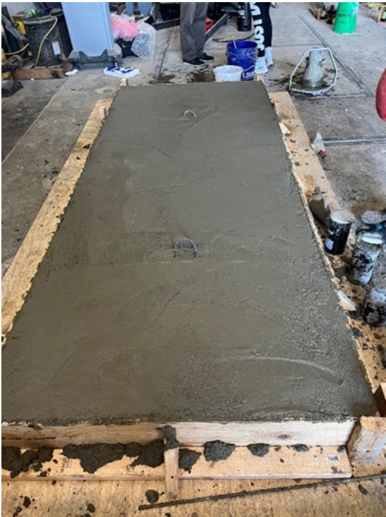
(c) Freshly Finished Concrete Surface
