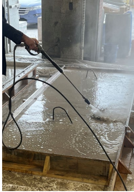
Figure 6.5 Removal of surface retarder using high-pressure water.
