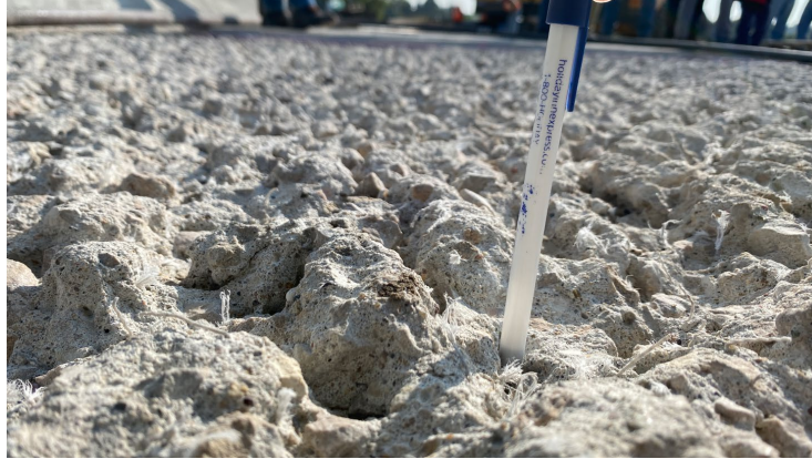
Figure C.1 Surface of bridge deck after hydro-demolition.
