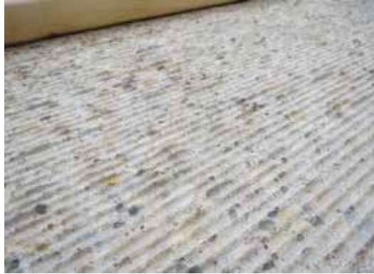
Figure 2.10 Deck surface after grinding (Haber et al., 2018).
