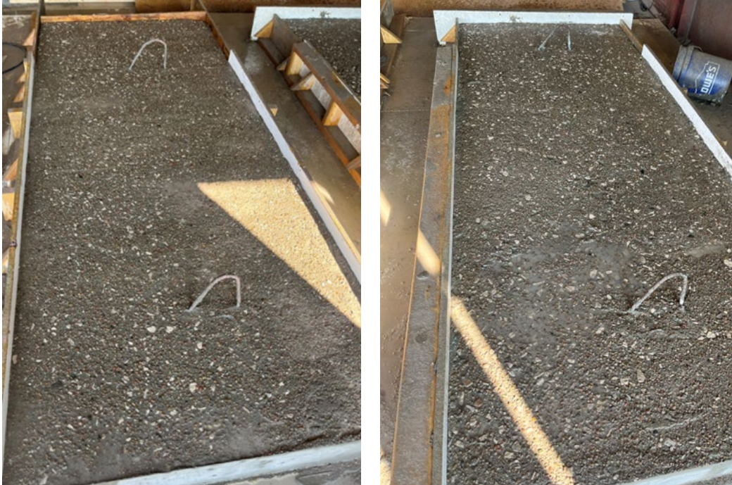
(a) Slab prepared with Master-Finish XR surface retarder (Pink) from Master Builders
