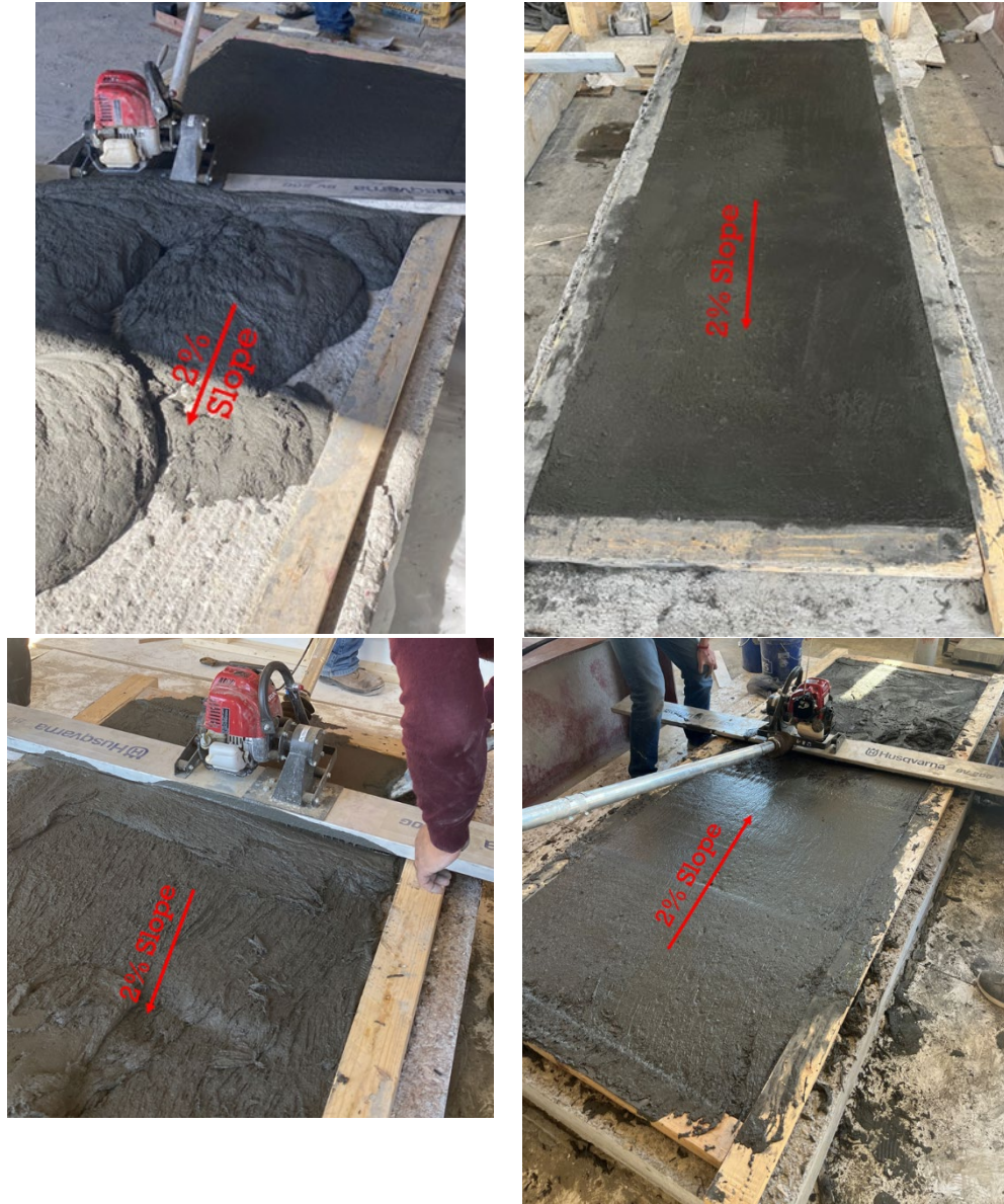
(a) During placement
