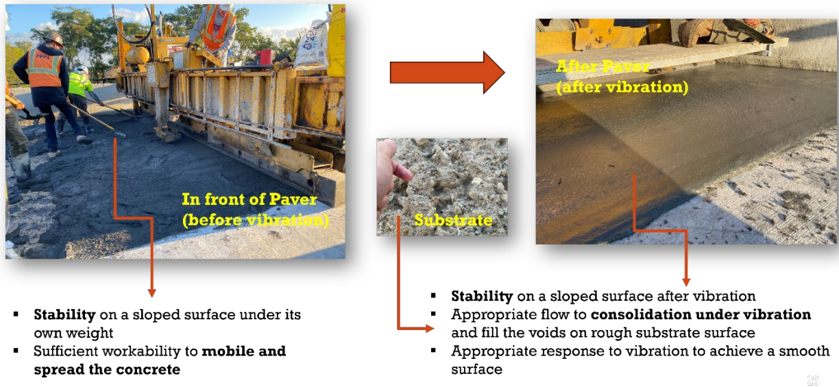
Figure 2.5 Thixotropic (overlay) UHPC workability characteristics.
