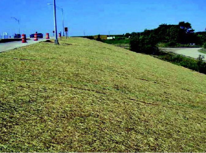
Pictured: Good Erosion Control Blanket installation.
