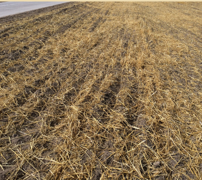
Pictured: Good installation of mulch
