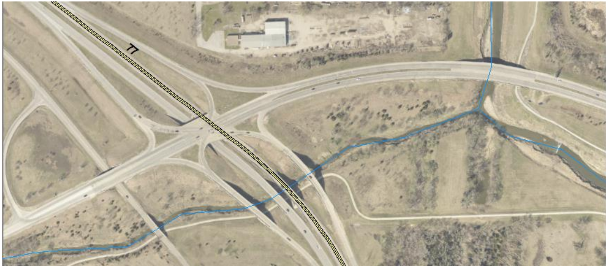
FIGURE 6. EXAMPLE OF STATE HIGHWAY INTERSECTION WITH WATER OF THE STATE
